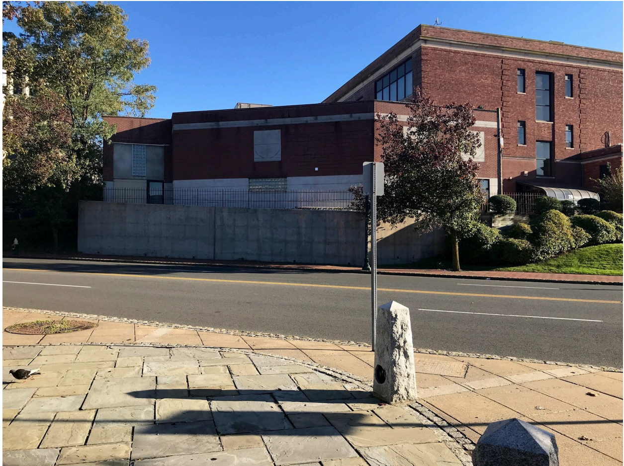
Valley Street Retaining Wall - from across the street
