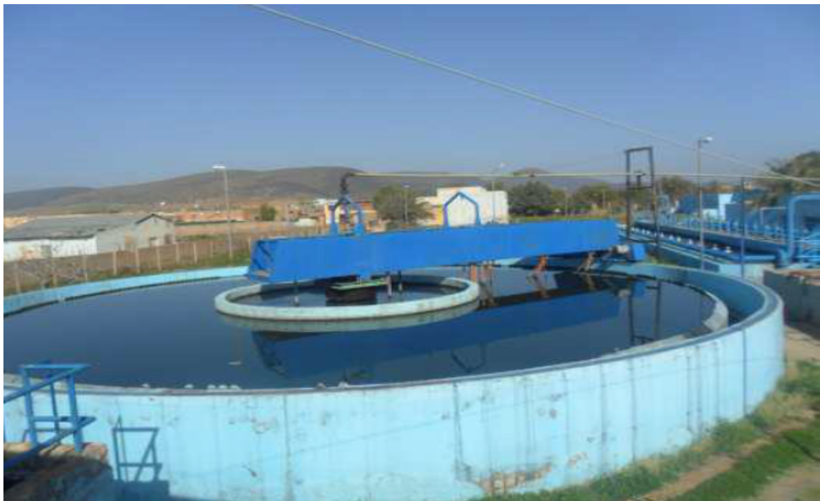
Figure 4. Clarifying flocculator.
