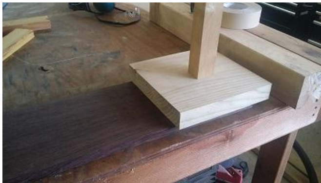
Figure 7 Where the riser and anchor will be placed. Note, the rails are missing from this picture and will be added later.
