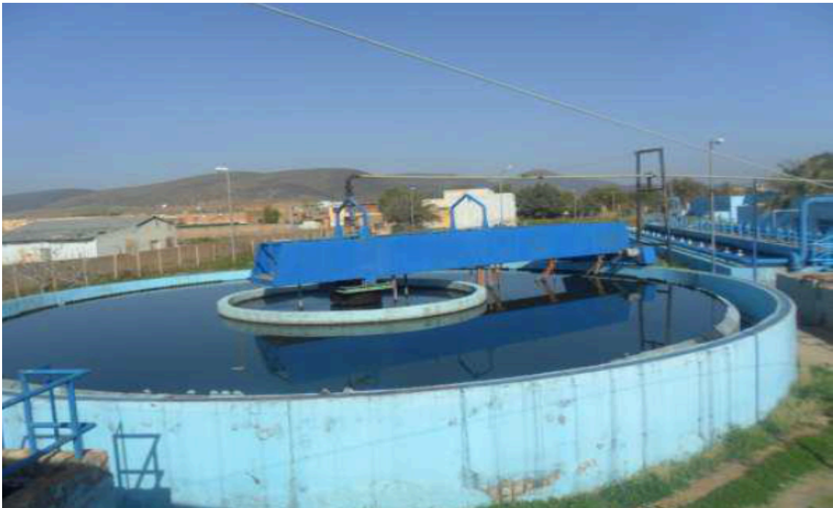
Figure 4. Clarifying flocculator.
