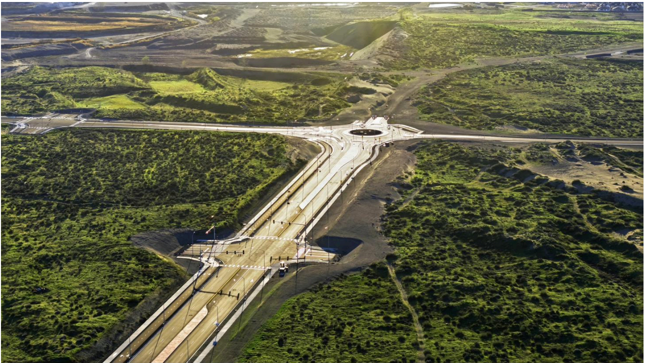
Newly constructed roundabout and road network serving the Riverbend Marketplace development.
