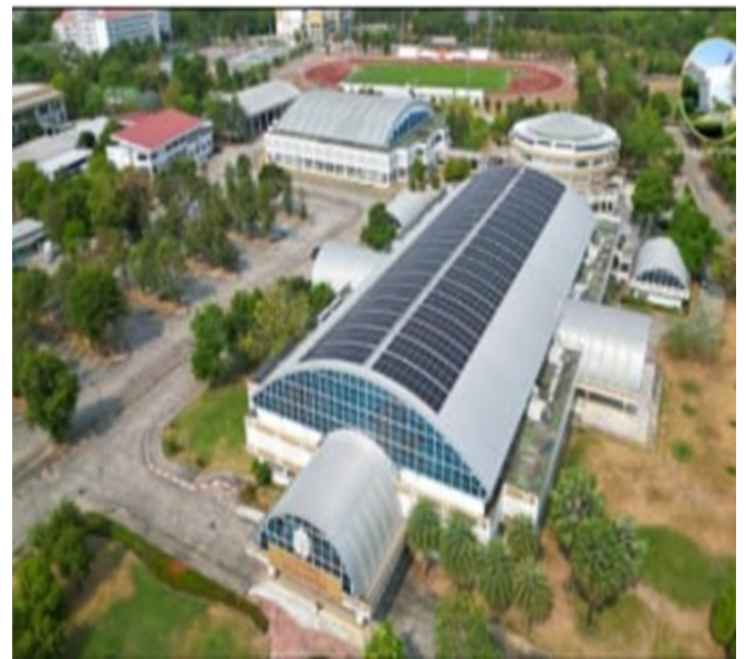
2. Solar Rooftop at Sisaket Rajabhat University
