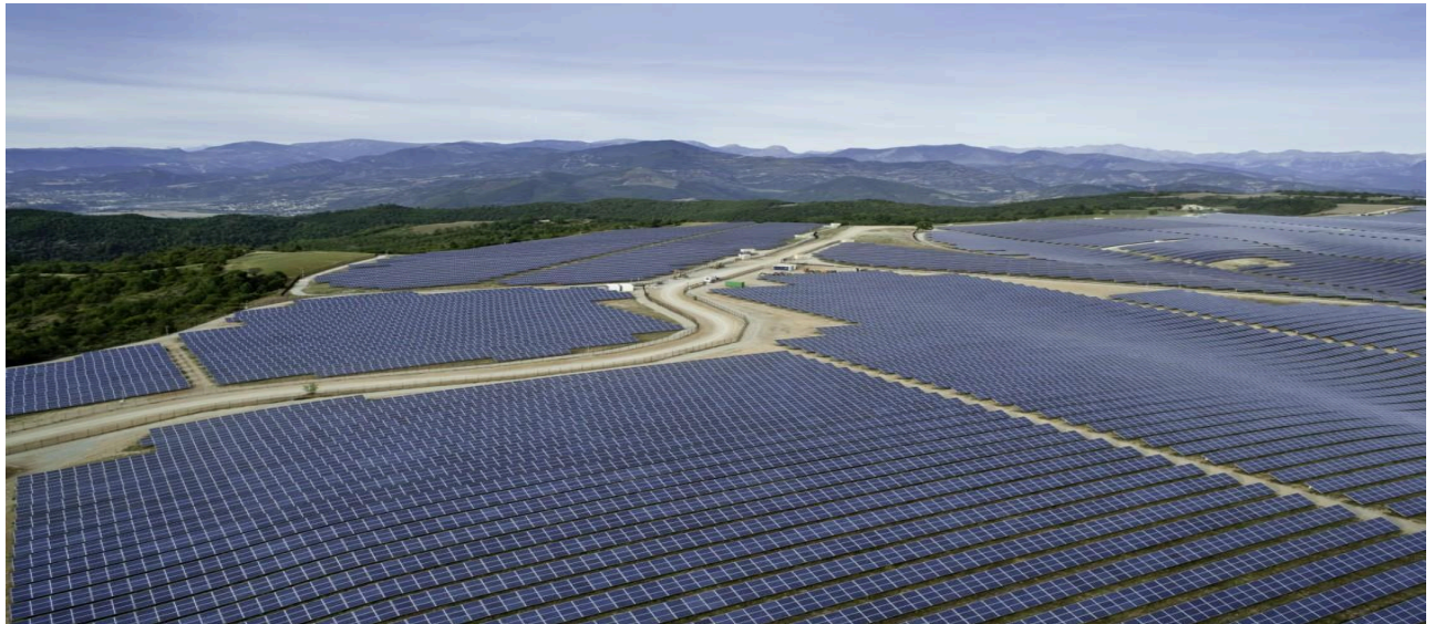
Figure.1.4 Photovoltaic solar power plant
