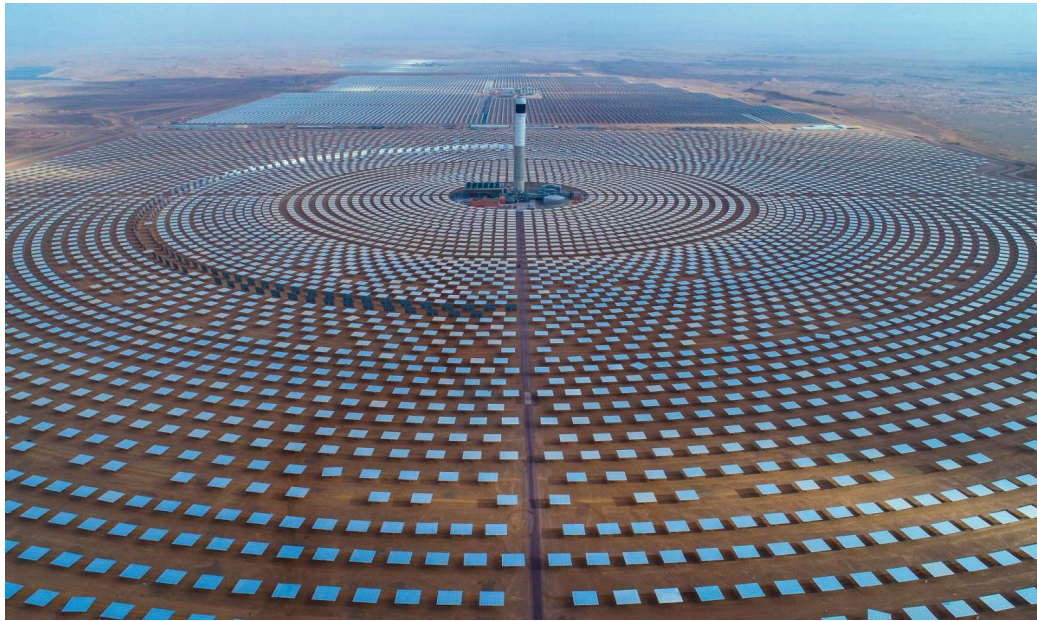
Figure.1.5 Concentrated Solar Power plant
