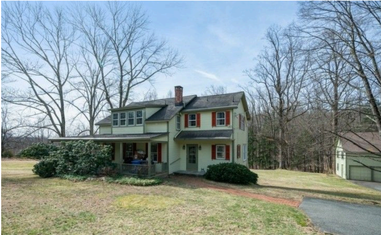
C. 1850s. East Jersey Cottage with 1970s additions. 2-story barn is also a contributing structure. Fieldstone foundation denotes the oldest part of the house.
