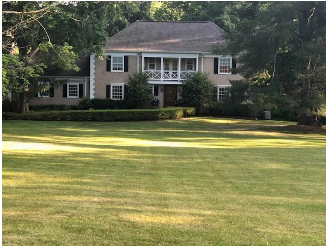
C. 1930 French Eclectic Revival. 2 ½ story manor house. Slate roof, brick chimneys. Garage does not contribute.
