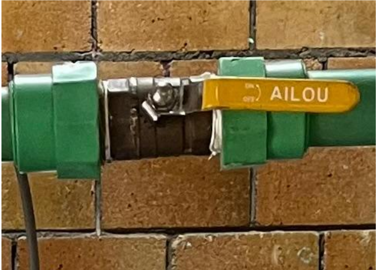
Fig3.11 Flow control valve.
