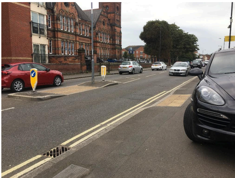
5 A road with heavy traffic (well above 5000 vehicles per day), uncontrolled crossing points and dangerous pavement parking
