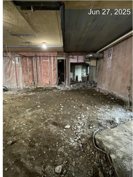
Kitchen Slab Removed
