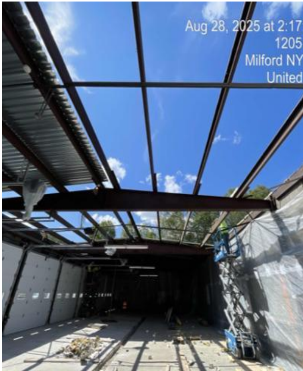
Bus Garage Roof Demo/Install
