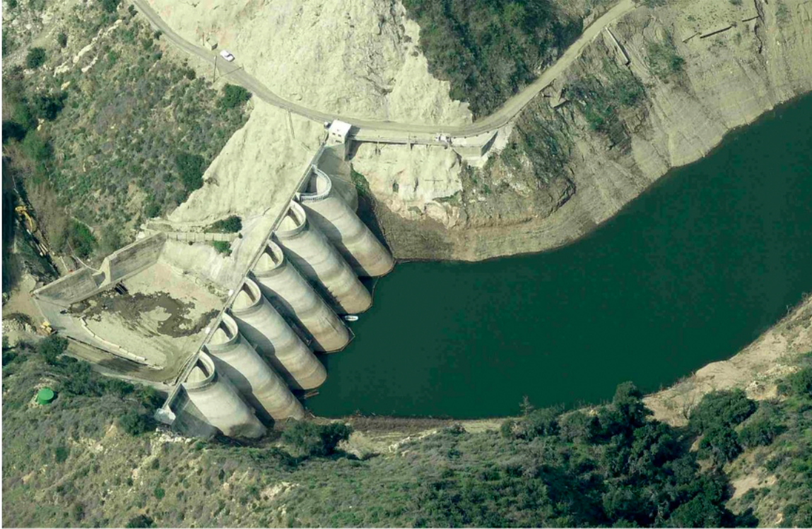
Figure 3: The six multiple arches of Big Dalton Dam. The original dam whose construction was abandoned is seen downstream of the current dam. 16
