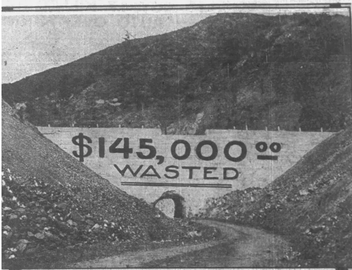
Figure 1: The core wall of the original partially constructed Big Dalton Dam that was abandoned. A road was built through this structure to facilitate construction of a new dam farther up the canyon. In this photo the amount of money that had already been spent was superimposed on the concrete wall. 17
