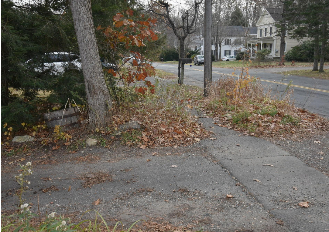
Driveway at 21 S. Main St., looking south
