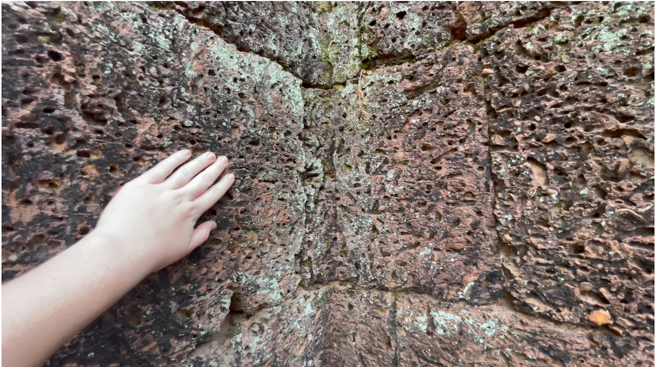
Image 5. Curved corner blockwork of the outer temple wall construction at Banteay Srei
