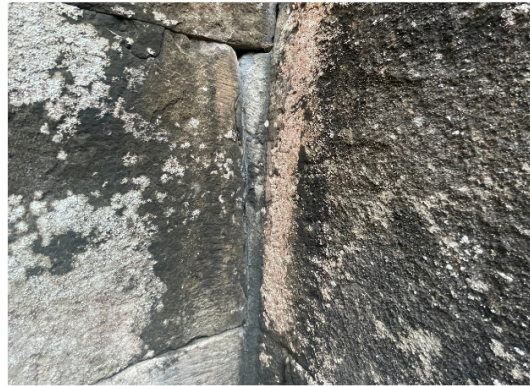
Curved Corner Blockwork
