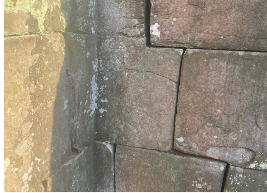
Curved Corner Blockwork
