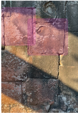
L-Shaped Blockwork
