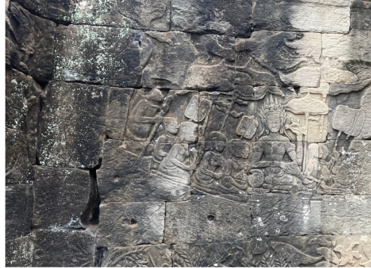
Curved Corner Blockwork
