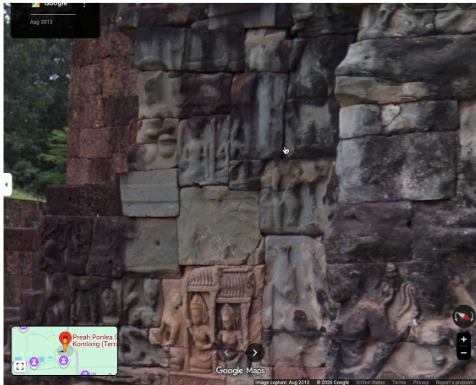
L-Shaped Blockwork
