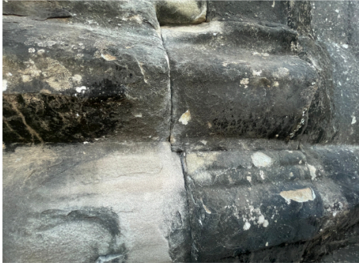
L-Shaped Blockwork
