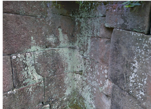
Curved Corner Blockwork
