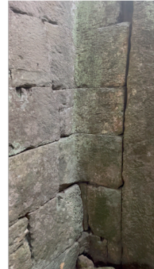
Curved Corner Blockwork
