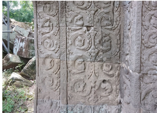
Curved Corner Blockwork
