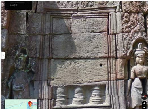
L-Shaped Blockwork
