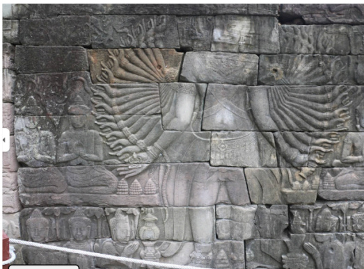
L-Shaped Blockwork
