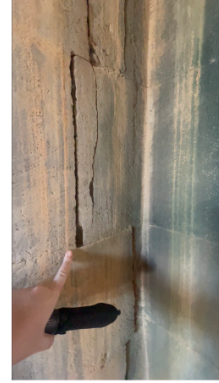
Curved Corner Blockwork
