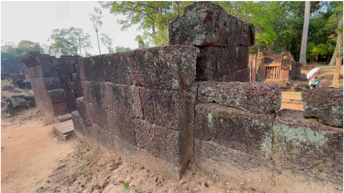
Image 6. Curved corner blockwork of the outer temple wall construction at Banteay Srei
