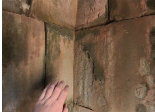
Curved Corner Blockwork
