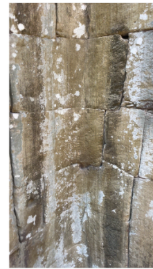
Curved Corner Blockwork
