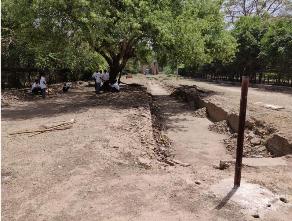
AFTER THE CLEANING WORK
