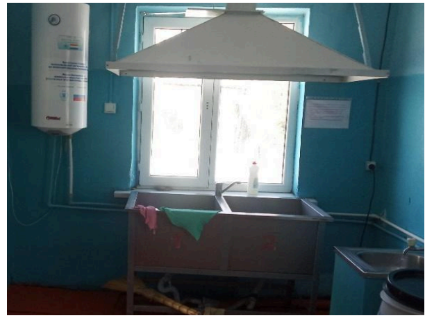
Fig.23, 24 - Local ventilation exhaust pump in the kitchen
