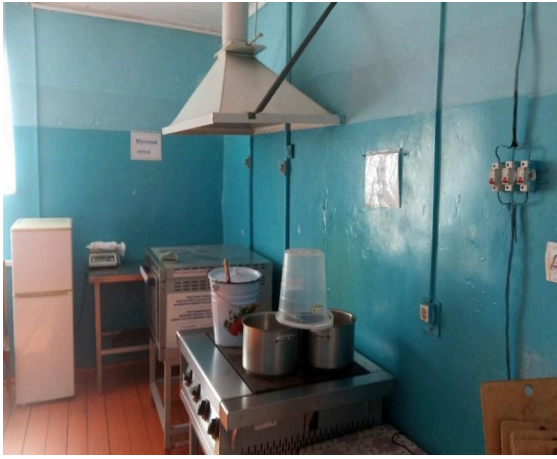
Fig.23, 24 - Local ventilation exhaust pump in the kitchen
