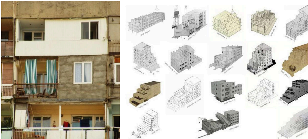
Illustration: (left) modification made to housing by residents to accommodate larger families. (right) Examples of Soviet housing typology
