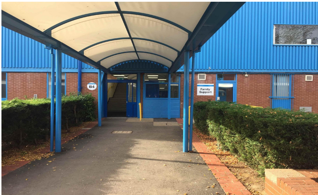
Figure 2: B4 Entrance to a building which has the following rooms:
