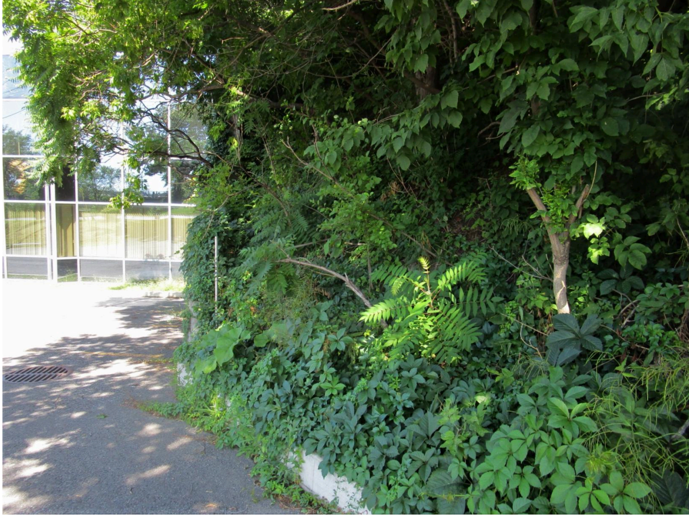
The beginning of “D” section near Avon showing office building built right to the base of the Falaise Arc
