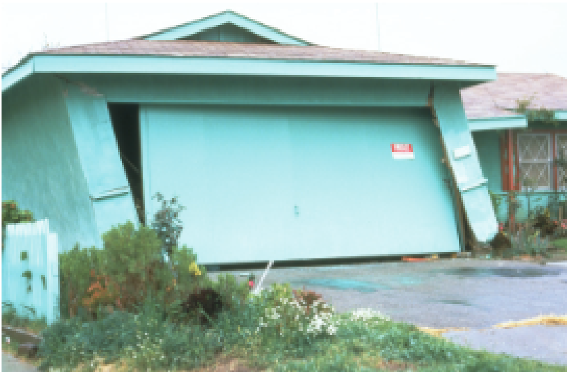
Figure 8-2 Earthquake damage at garage door opening in a one-story house (from ATC, 2002).
