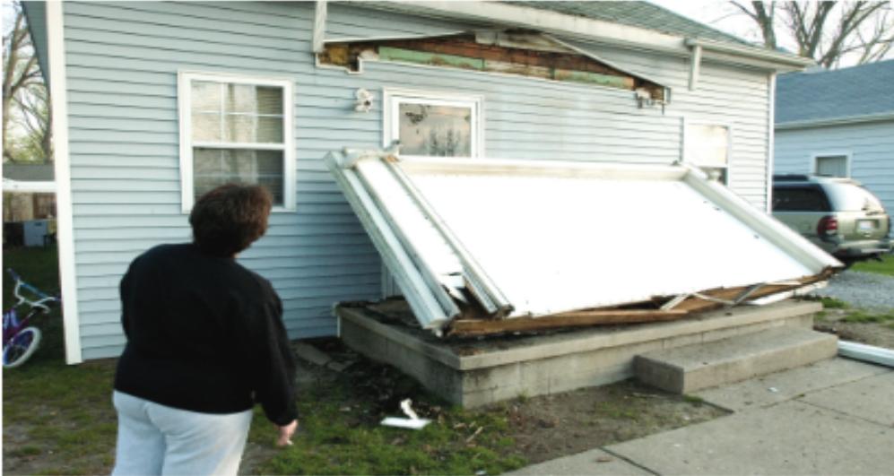
Figure 7-9 Porch roof broken off (and repositioned) in Mt. Carmel, Illinois, by the Richter magnitude 5.2 Mt. Carmel Earthquake in 2008. (Photo credit: Associated Press/Daniel R. Patmore)
