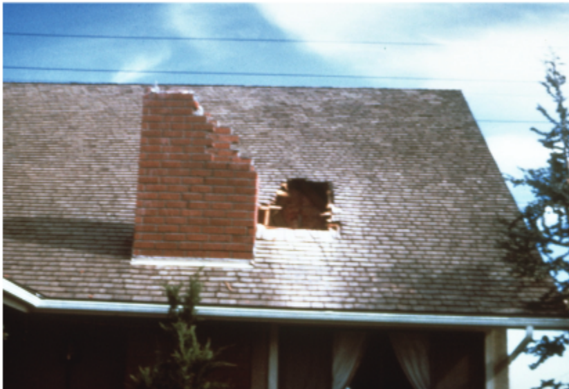
Figure 7-2 Masonry debris from an unreinforced chimney has fallen through the roof into the living spaces (from ATC, 2002).
