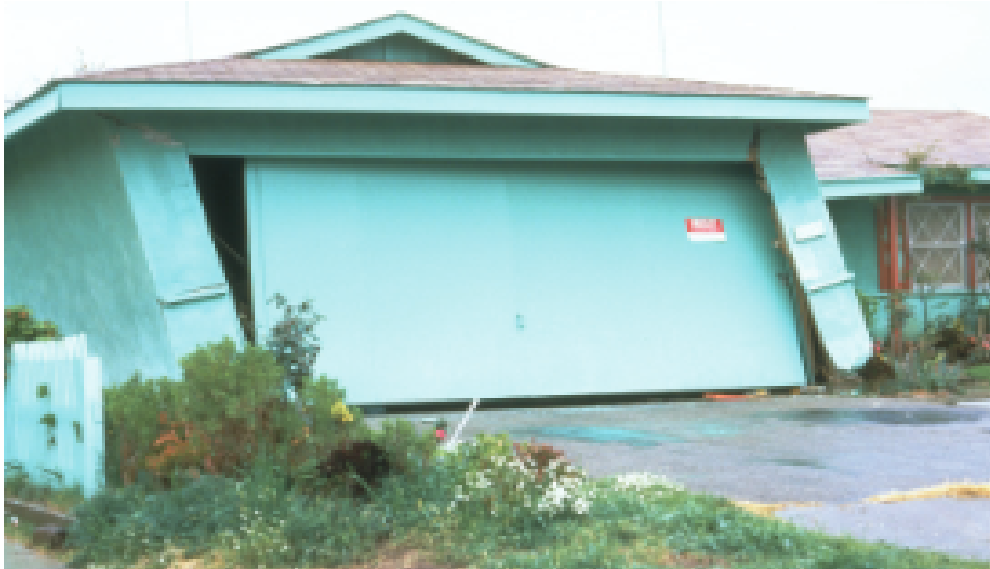
Figure 8-2 Earthquake damage at garage door opening in a one-story house (from ATC, 2002).
