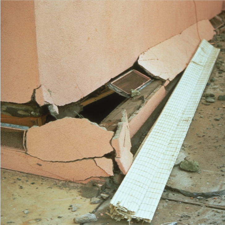
Figure 2-5 Typical earthquake damage to a cripple-wall house (from ATC, 2002).
