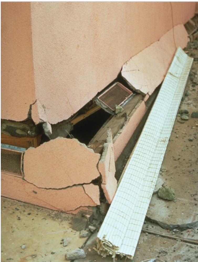
Figure 2-5 Typical earthquake damage to a cripple-wall house (from ATC, 2002).
