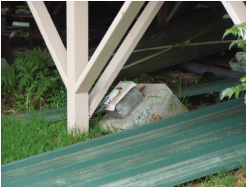
Figure 2-17 Earthquake-damaged perimeter post-and-pier foundation. The diagonally-braced post has overturned the shallow-founded concrete pier footing (from ATC, 2002).
