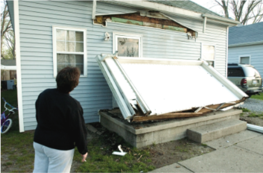
Figure 7-9 Porch roof broken off (and repositioned) in Mt. Carmel, Illinois, by the Richter magnitude 5.2 Mt. Carmel Earthquake in 2008. (Photo credit: Associated Press/Daniel R. Patmore)
