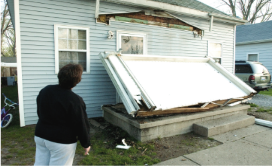
Figure 7-9 Porch roof broken off (and repositioned) in Mt. Carmel, Illinois, by the Richter magnitude 5.2 Mt. Carmel Earthquake in 2008. (Photo credit: Associated Press/Daniel R. Patmore)
