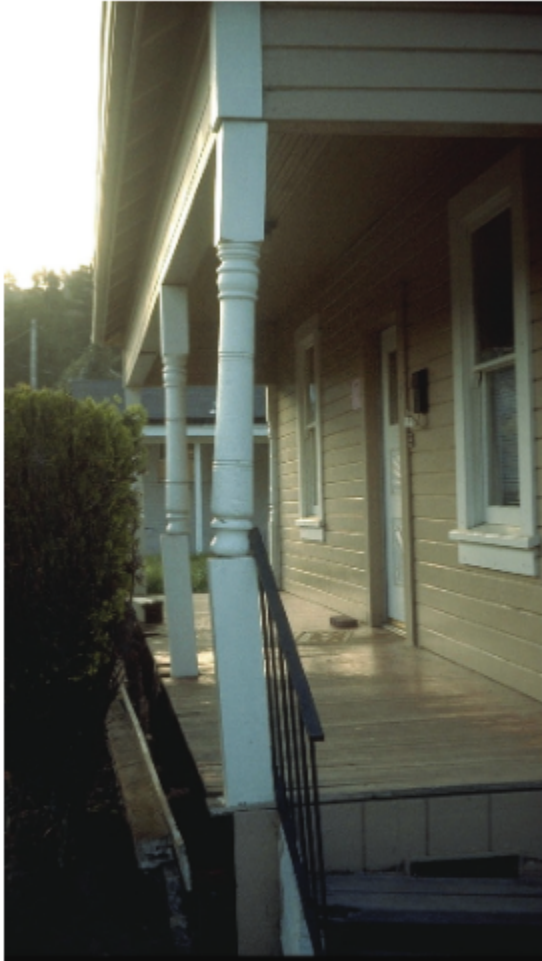
Figure 7-14 Failure of a porch roof support post by hinging at the middle (from ATC, 2002).
