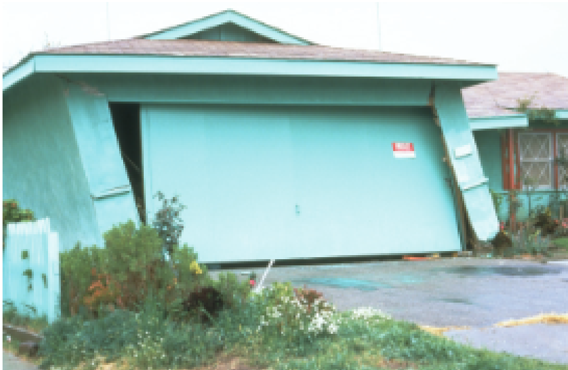
Figure 8-2 Earthquake damage at garage door opening in a one-story house (from ATC, 2002).
