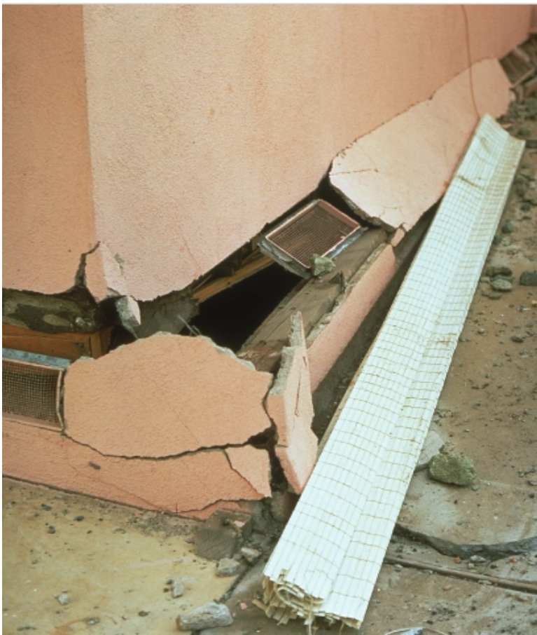
Figure 2-5 Typical earthquake damage to a cripple-wall house (from ATC, 2002).
