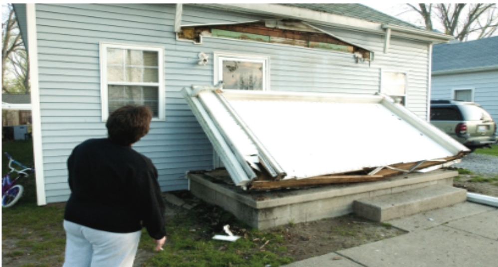
Figure 7-9 Porch roof broken off (and repositioned) in Mt. Carmel, Illinois, by the Richter magnitude 5.2 Mt. Carmel Earthquake in 2008. (Photo credit: Associated Press/Daniel R. Patmore)
