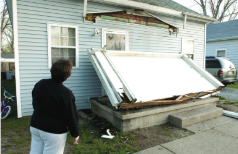
Figure 7-9 Porch roof broken off (and repositioned) in Mt. Carmel, Illinois, by the Richter magnitude 5.2 Mt. Carmel Earthquake in 2008. (Photo credit: Associated Press/Daniel R. Patmore)
