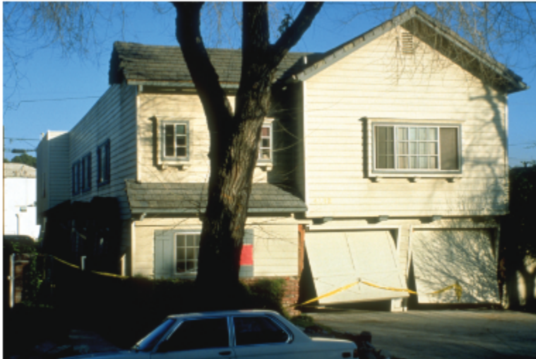
Figure 2-10 Damage and racking displacement to the right in the first floor walls of a two-story slab-on-grade house (from ATC, 2002).
