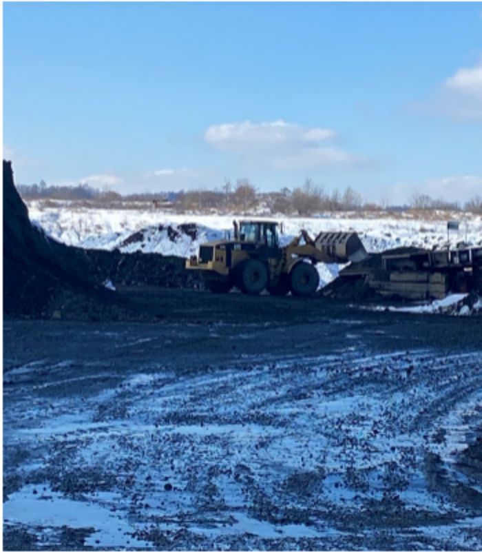
Waste coal is put into piles at the Grant Town Power Plant last week. | Scott Waldman/E&E News
