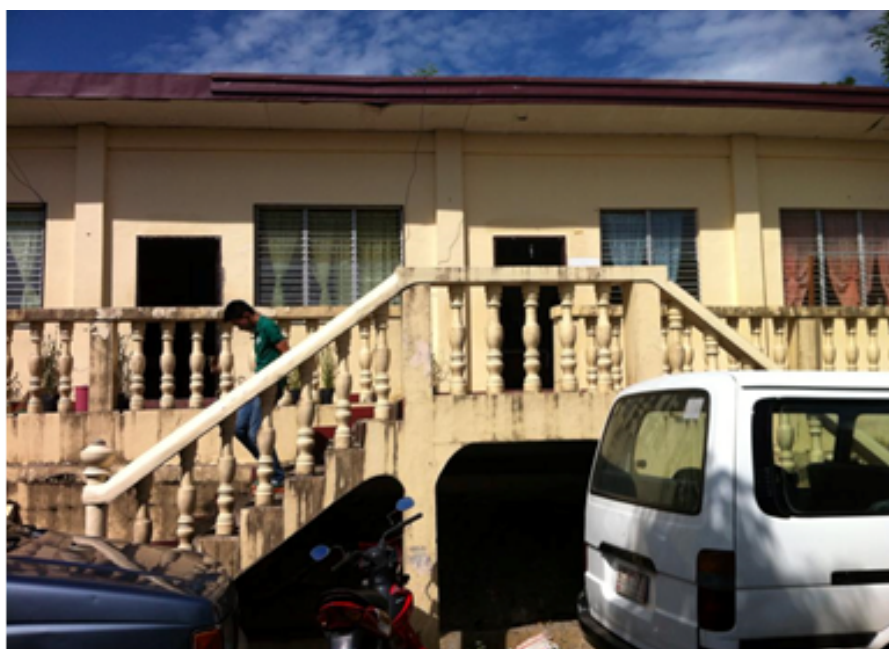
The Old Student Center That Was Demolished
