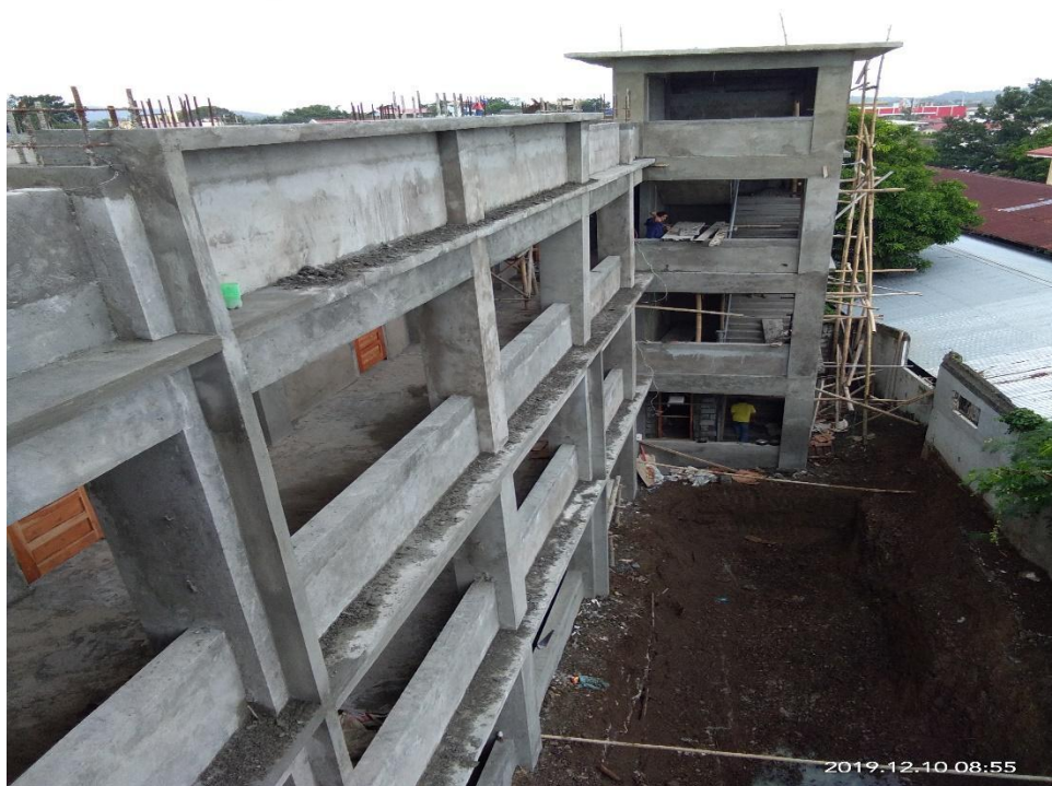
The Three-storey Nine-classroom Building Being Constructed
