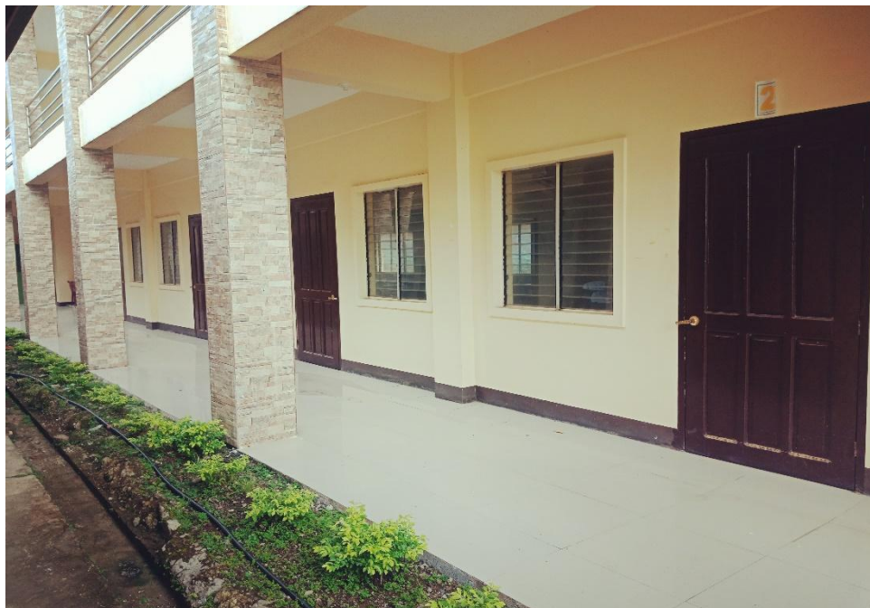
The ground floor of the CM new building houses 2 classrooms
