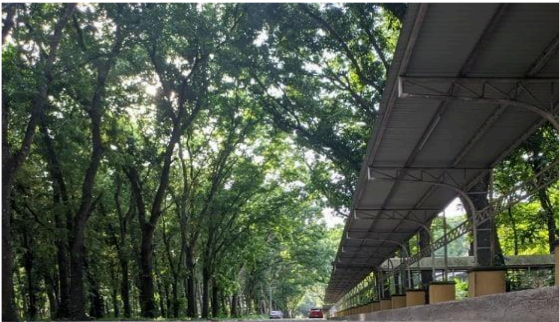
Well Built pathways with roofing
