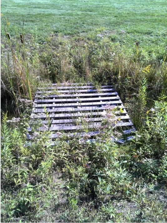
S7-24: End of Ditch
