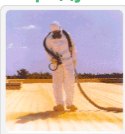
▲ Spray Coat Insulation
