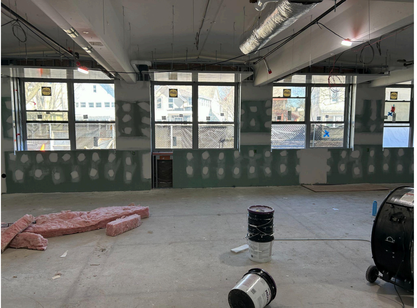
Windows are complete, along with mudding the sheetrock seams in the classrooms on the Walnut Street side of the building.
