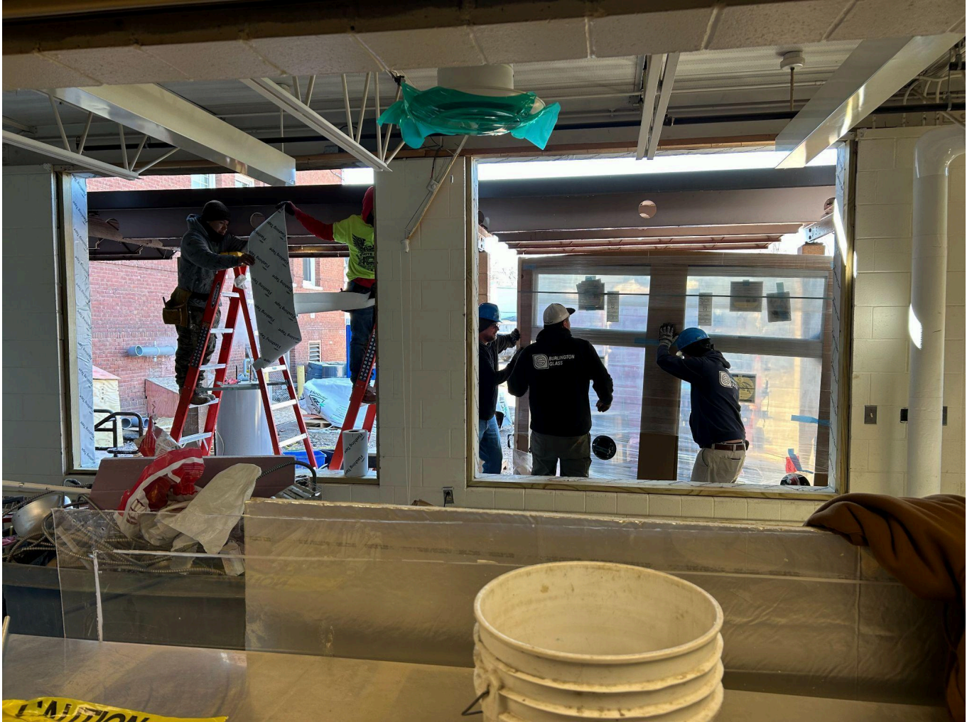
Out with the old and in with the new. Burlington Glass workers are shown installing the new energy efficient windows, while workers prep the existing window (on the left side) opening for the new windows in the cafeteria.
