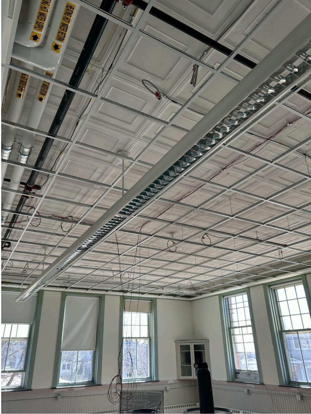
The Framing Contractor has finished the installation of the ceiling grid on the first floor in the 1904 wing of the building.
