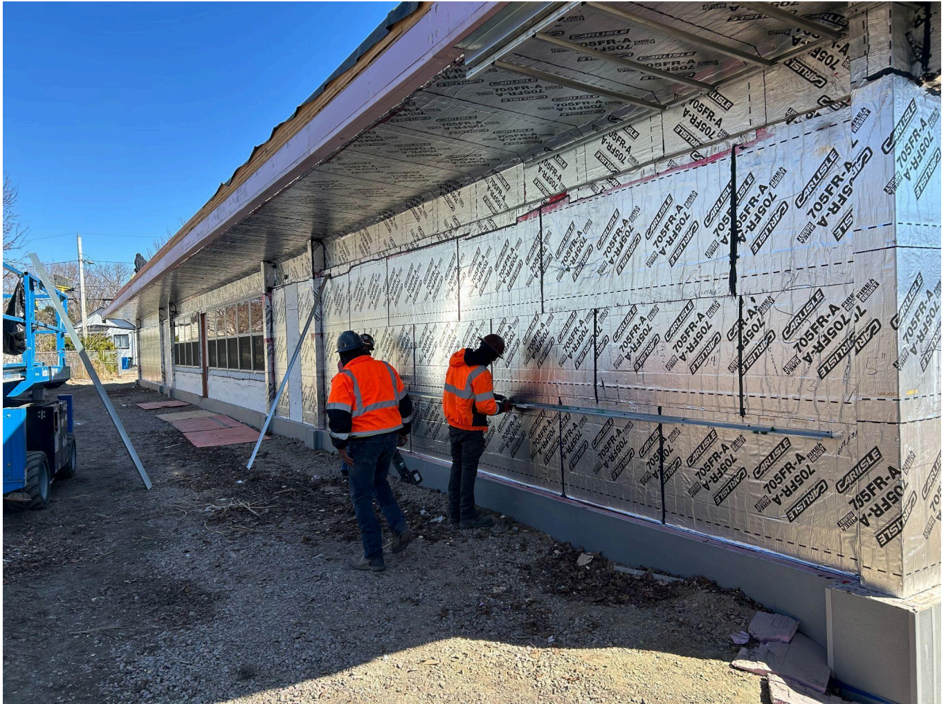
The North side of the 1965 wing of the building has received the vapor barrier and the new roof edge.
