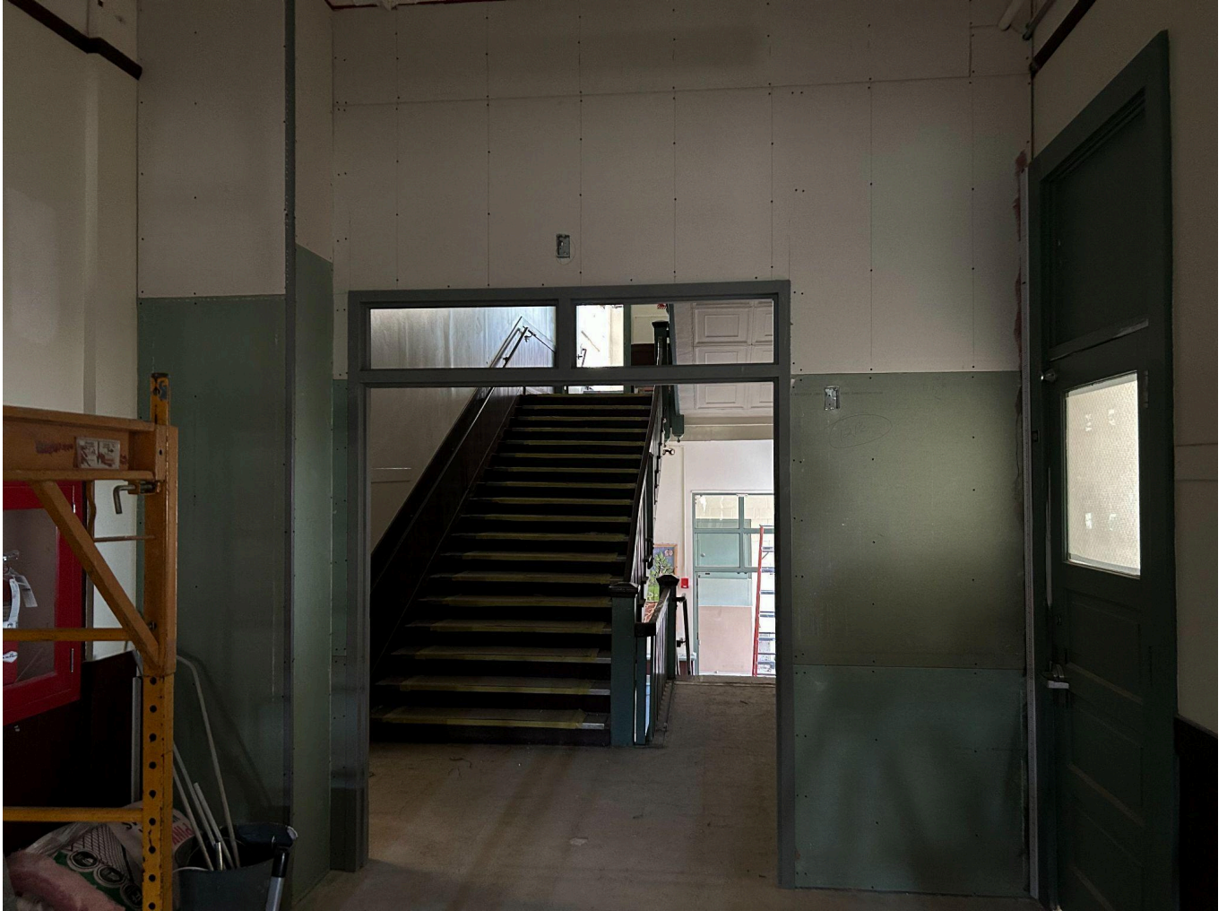
The Framing Contractor has installed the sheetrock on the wall framing the new doorway on the First Floor in the 1904 wing of the building.
