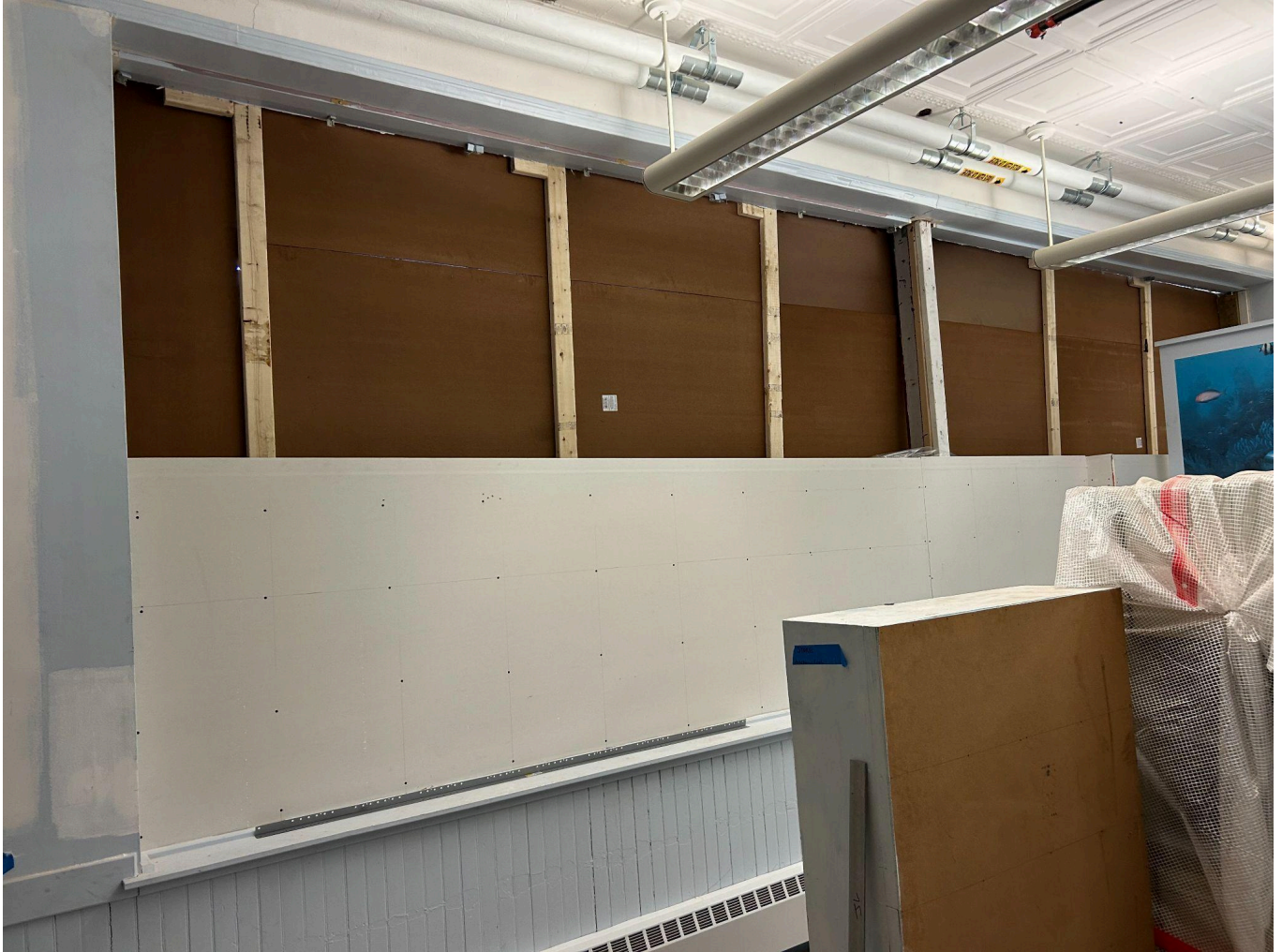
The Windows in the Dental Suite and Nurses Office will be changed out as well. This is showing the removal of the old windows, along with the new framing that is associated for the new windows.
