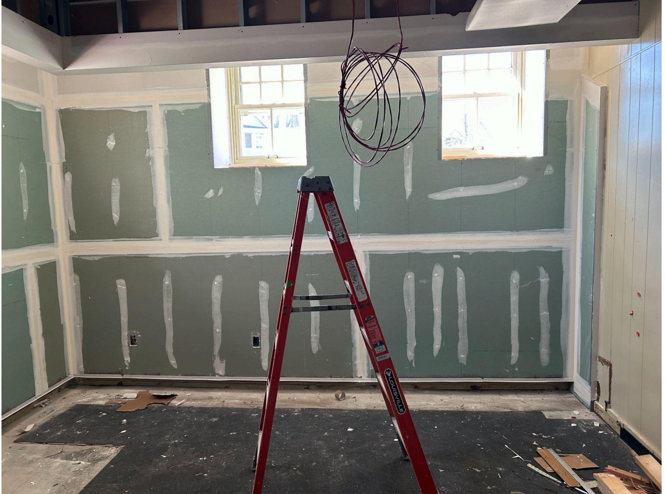
The Framing Contractor has finished the sheetrock and the tapers are starting the mudding process on the walls in the Basement in the 1904 wing of the building.
