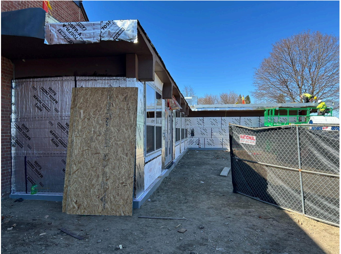
The exterior of the building getting the vapor barrier installed along with working on updating the roof edge on the Walnut Street side of the 1965 wing of the building.
