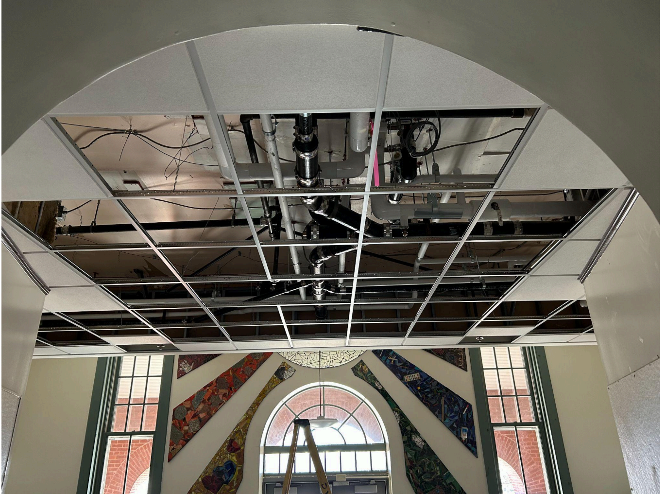
The Framing Contractor has framed up the new ceiling grid in the front Lobby in the 1904 wing of the building.
