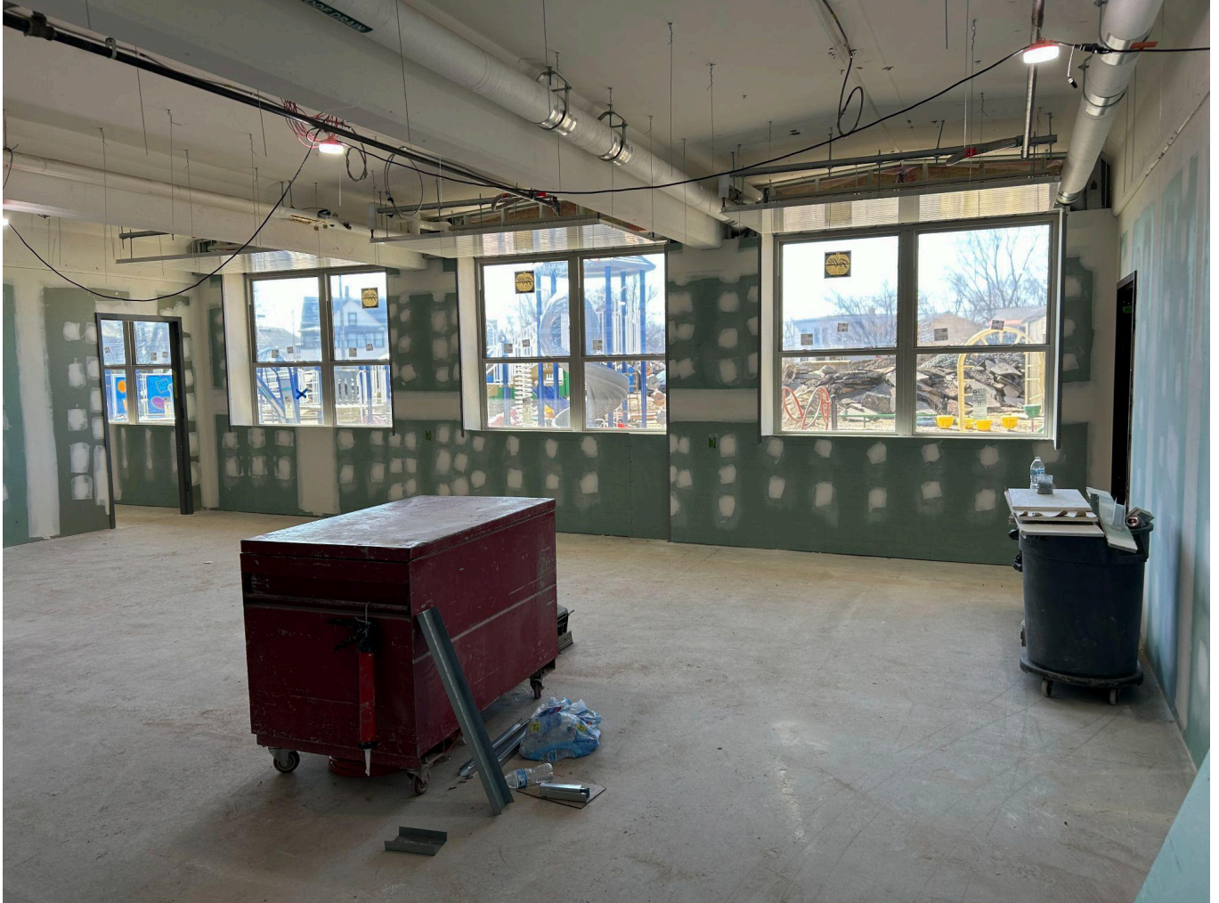
Windows are complete, along with mudding the sheetrock seams in the classrooms on the Spring Street side of the building.
