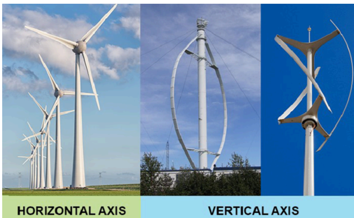
Figure1-3: Horizontal versus vertical axis wind turbines.
