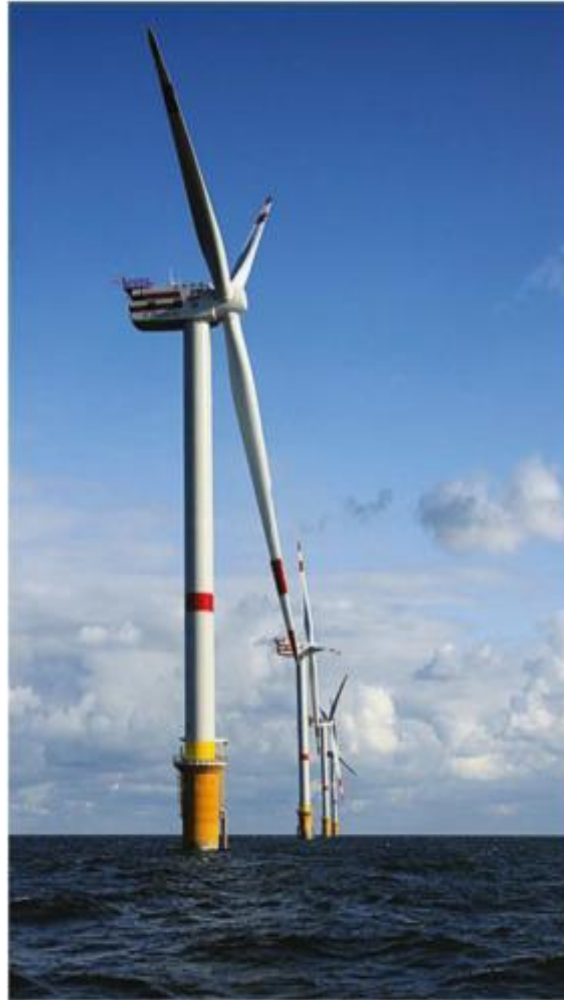
Figure 1-5: An offshore wind farm with three bladed horizontal axis wind turbines.
