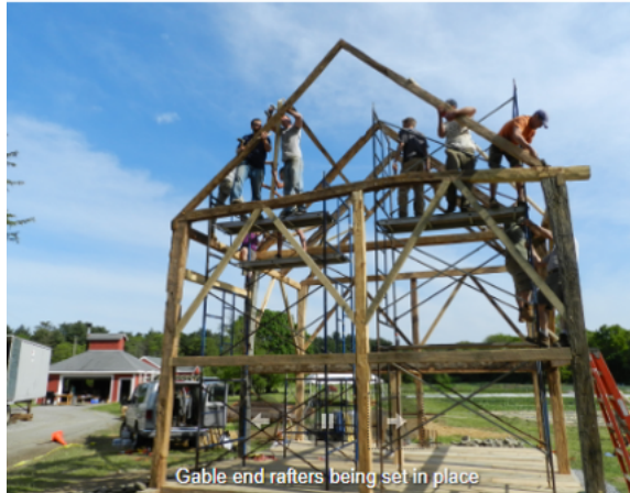
Gable end rafters being set in place
