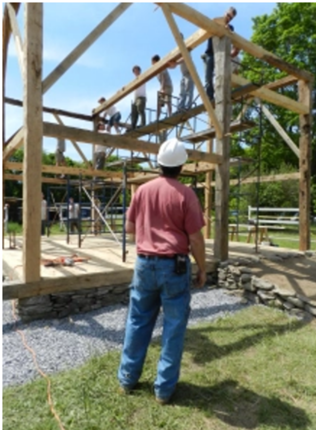
Gable end rafters being set in place
