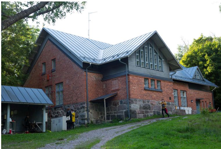
The main building of the island
