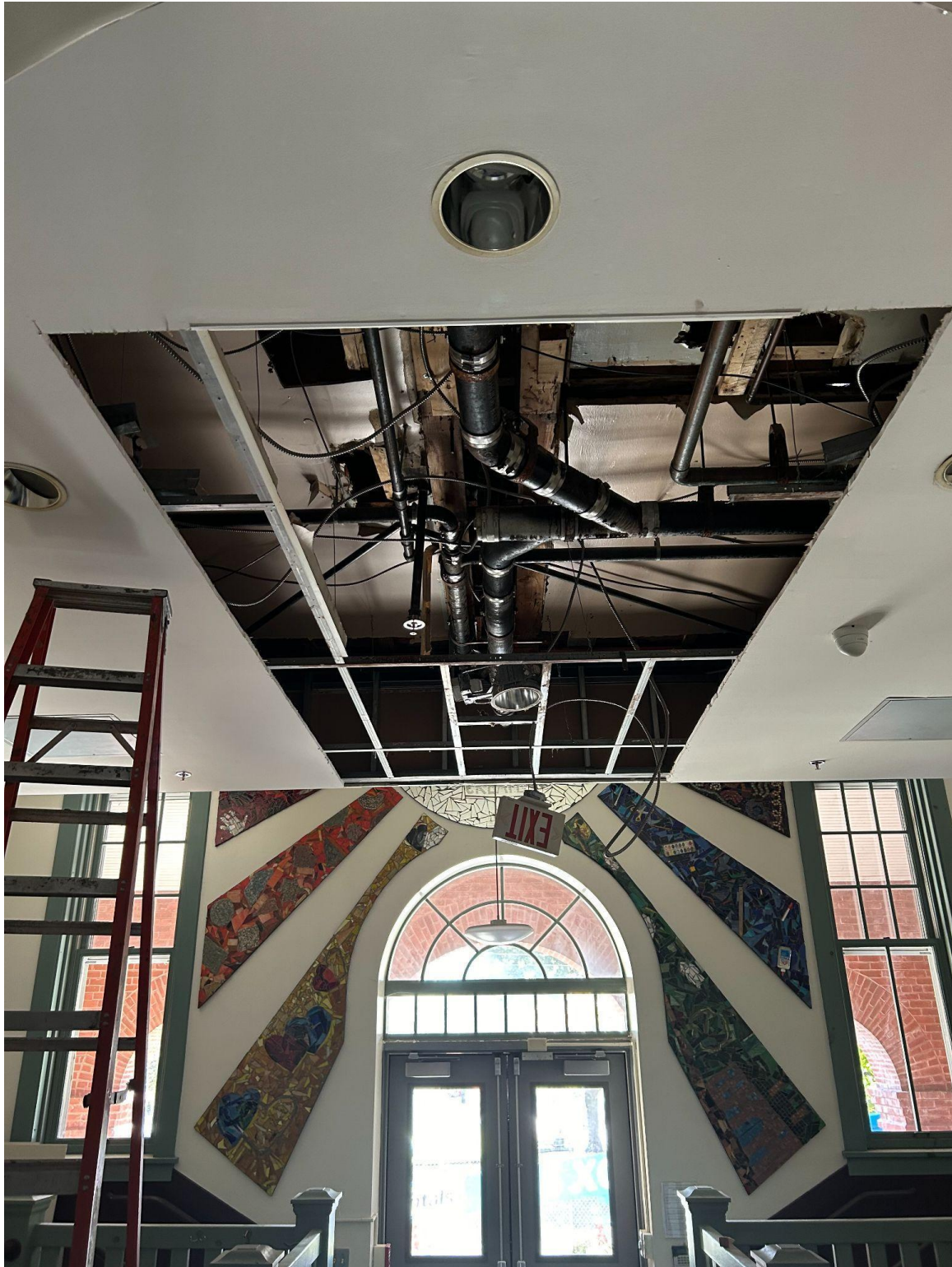
A picture showing the existing sanitary sewer piping which is in the ceiling of the 1904 wing of the building's Lobby. This piping will get modified to accommodate the locations for the new plumbing fixtures.
