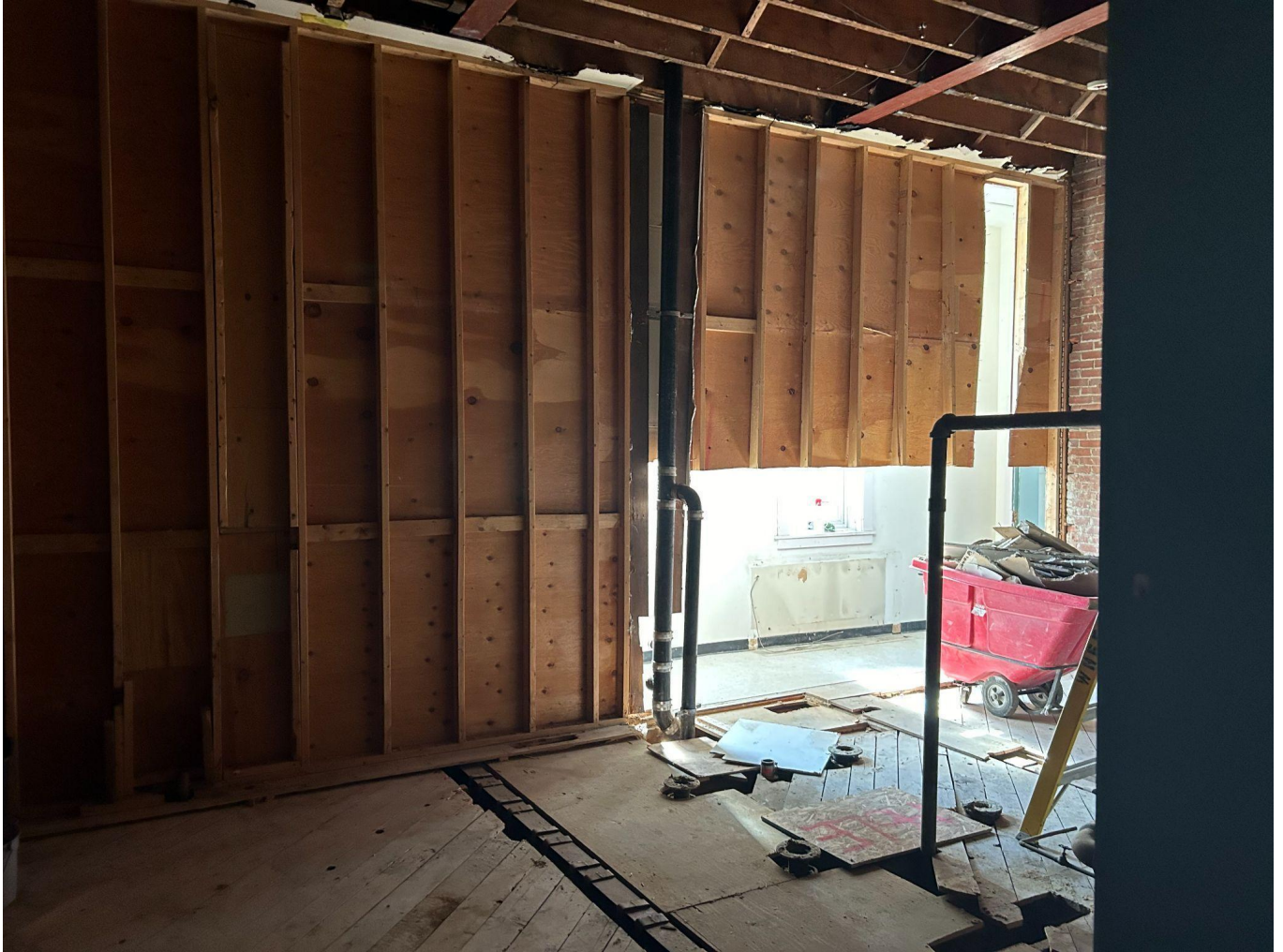
The start of demolition on the second floor existing gang bathrooms in the 1904 wing of the building.
