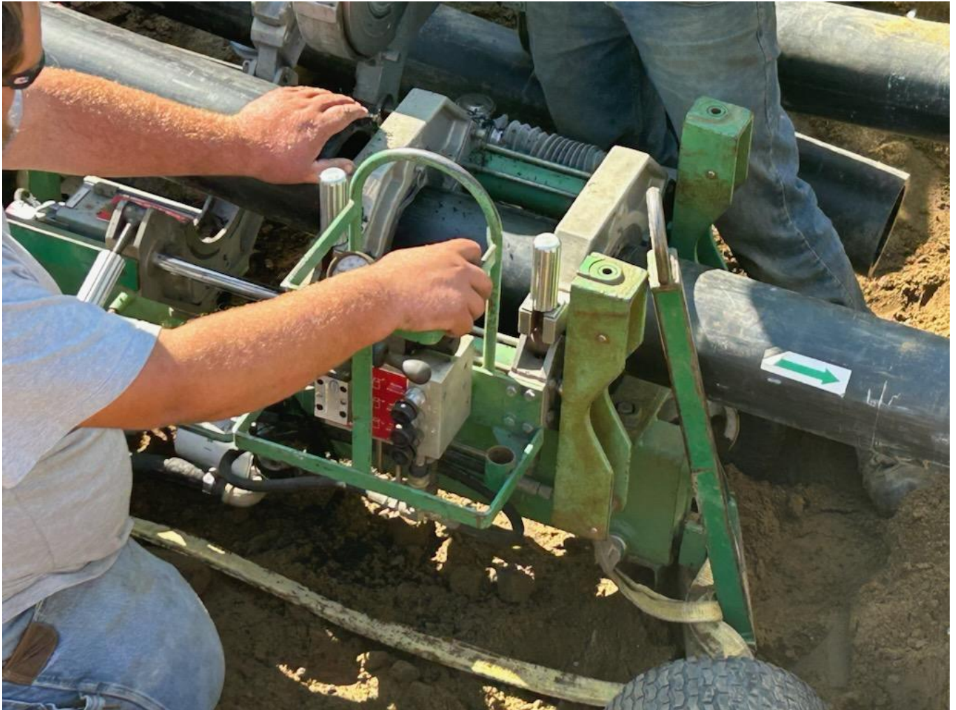
A Manosh worker is making up one of the last welded piping joint on the main geothermal piping coming from the vault that then goes into the building.
