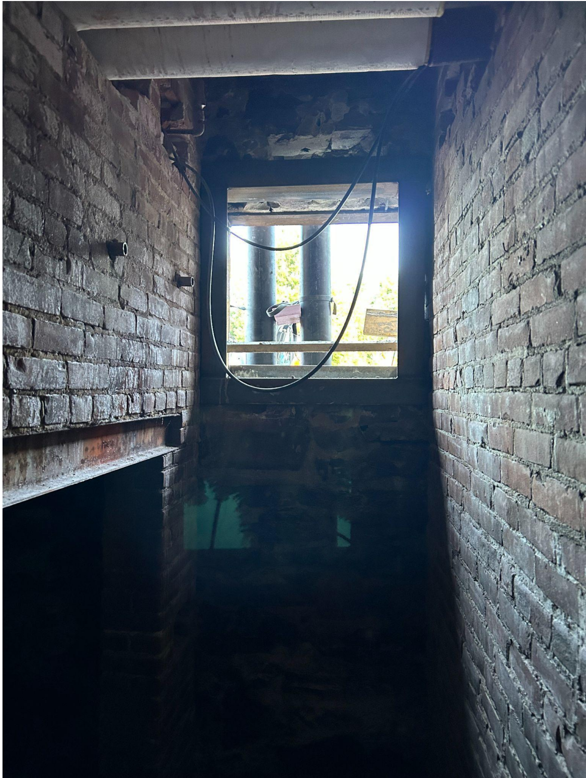
The hole in the building where the geothermal piping and the electrical conduits will be entering the building in the 1904 wing of the building in the basement.
