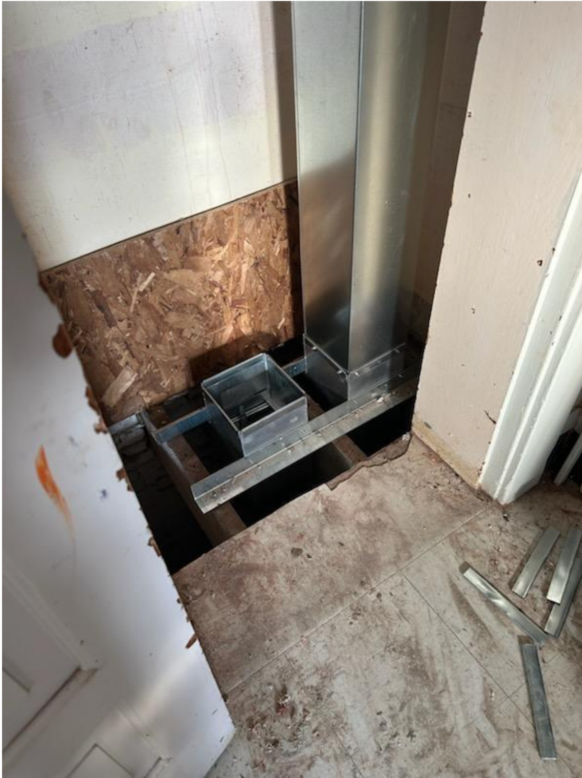
A picture showing ductwork being installed that will go from the basement up and into Attic space of the 1904 wing of the Building.
