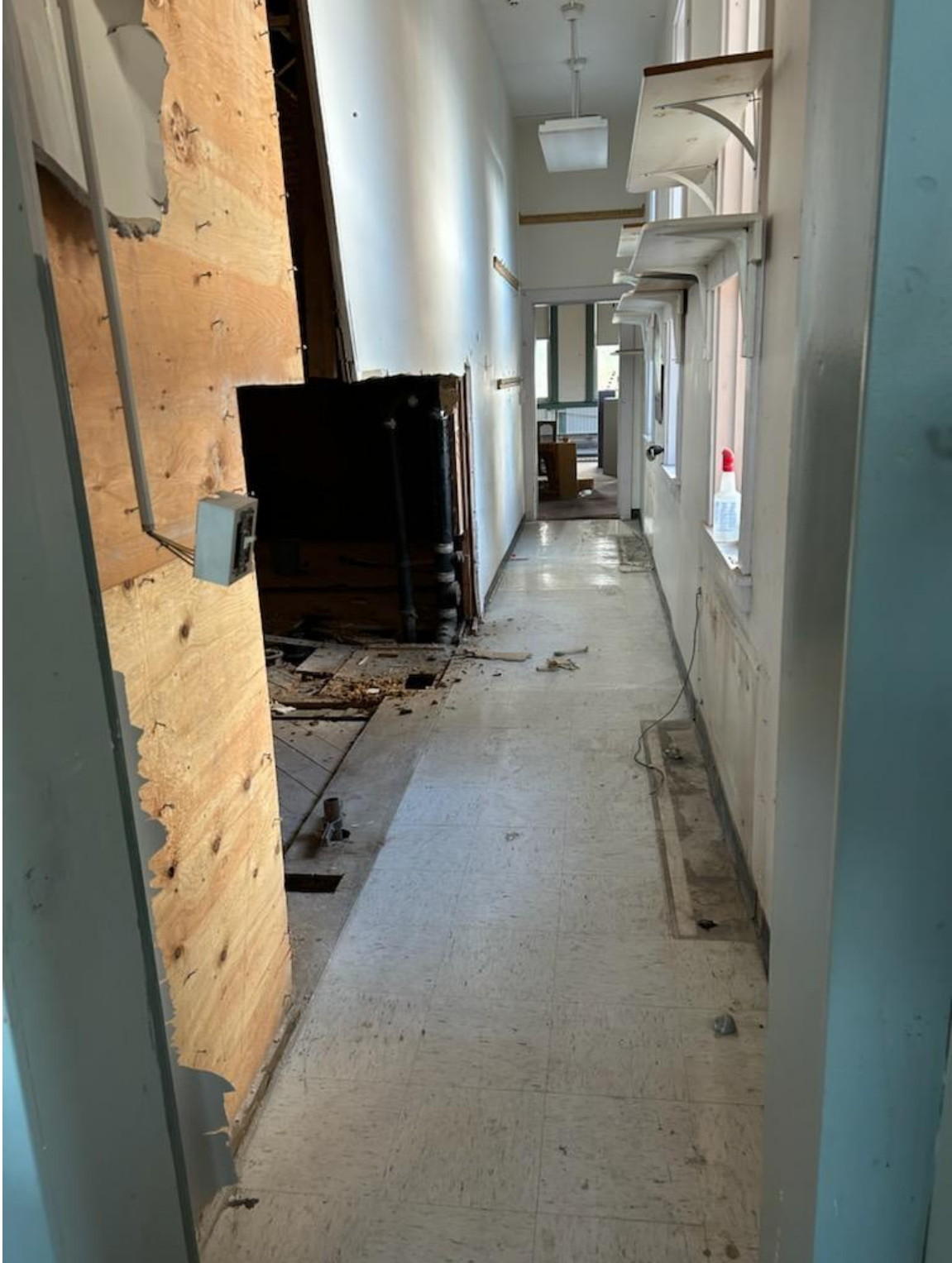
The backside view of the demolition of the second floor gang bathrooms in the 1904 wing of the building.
