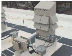
Above: Installed disconnects on VRF units on section B Roof.
