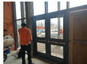
Above: Door installation in vestibule v101 main entrance.
