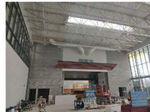
Above: Installed a screen over the return air duct at the stage area.
