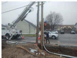
Above: Installed four 4" conduits for internet and communications.
