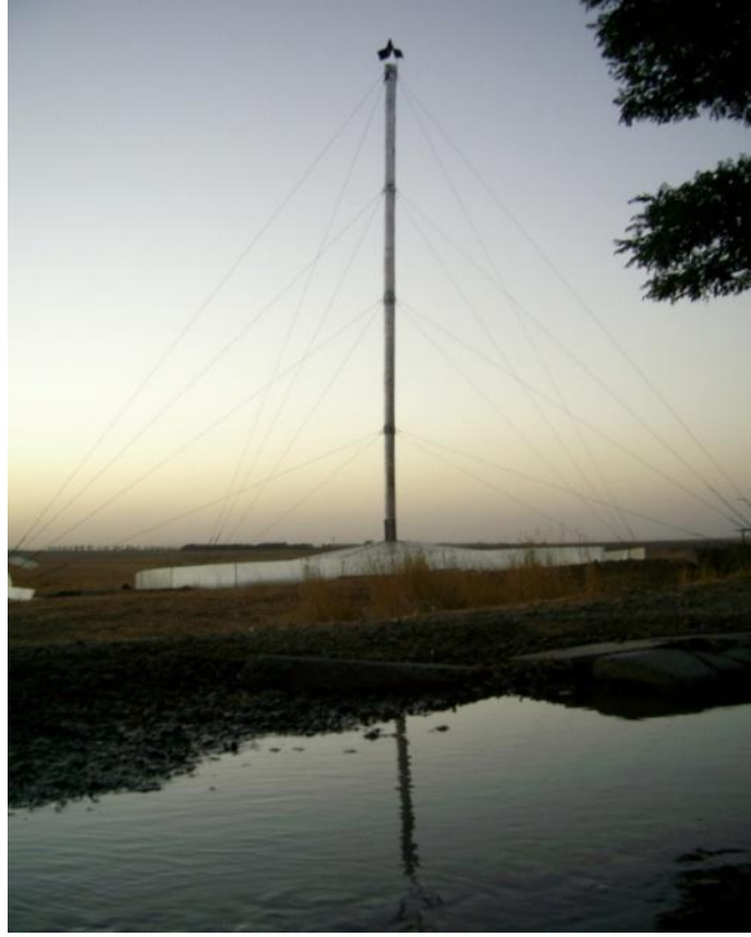
Figure 2-2: Zanajn solar chimney power plant.
