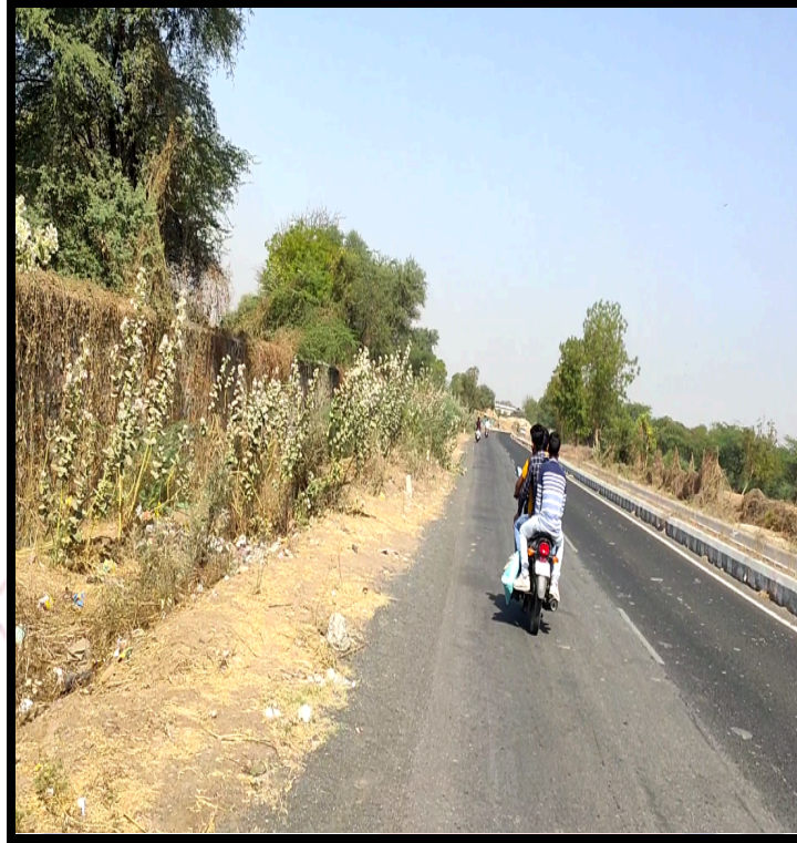
Figure 30 Shoulder width is not provided, guard rails for safety against trees is not provided and uneven road surface
