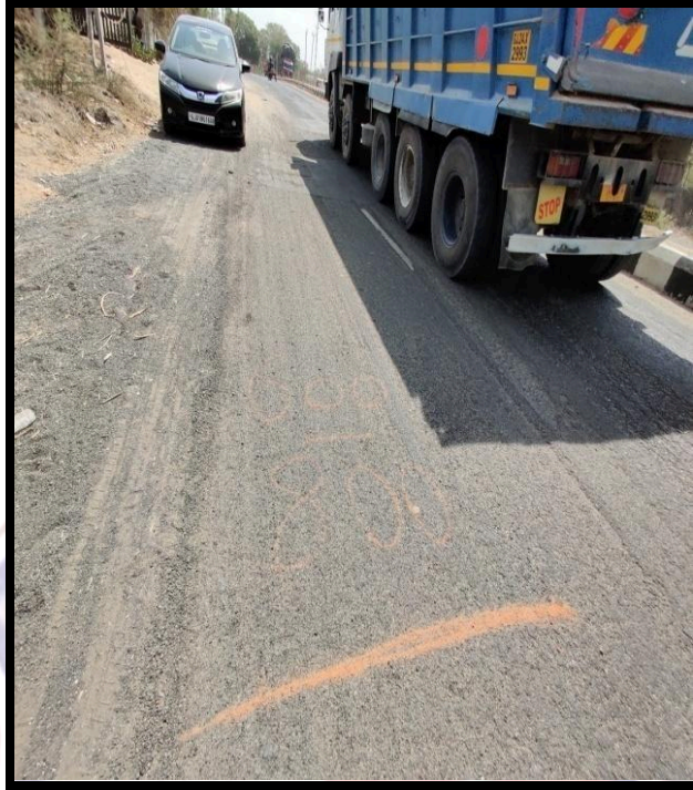
Figure 32 Wrong side moving vehicles, loose gravel on side of the road and no shoulder width provided
