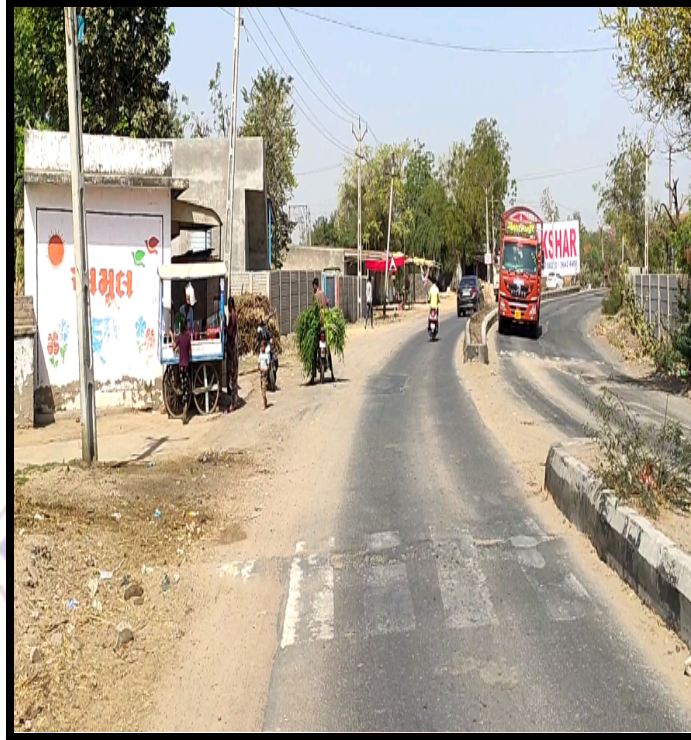
Figure 36 Poorly maintained road reducing road width, due to absence of shoulder width vehicles are parked unevenly on road side causing obstruction to moving traffic, no center line is provided and damaged median
