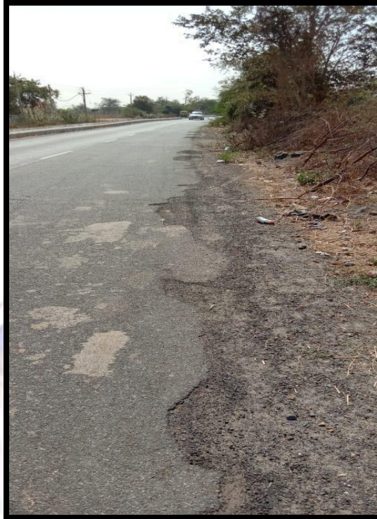
Figure 18 No shoulder width is provided, no fences are provided for safeguard against trees and turning movement
