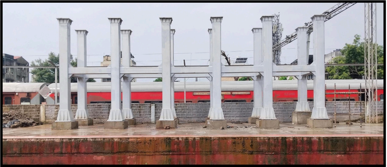
Improvement to FOB (Work in progress)
