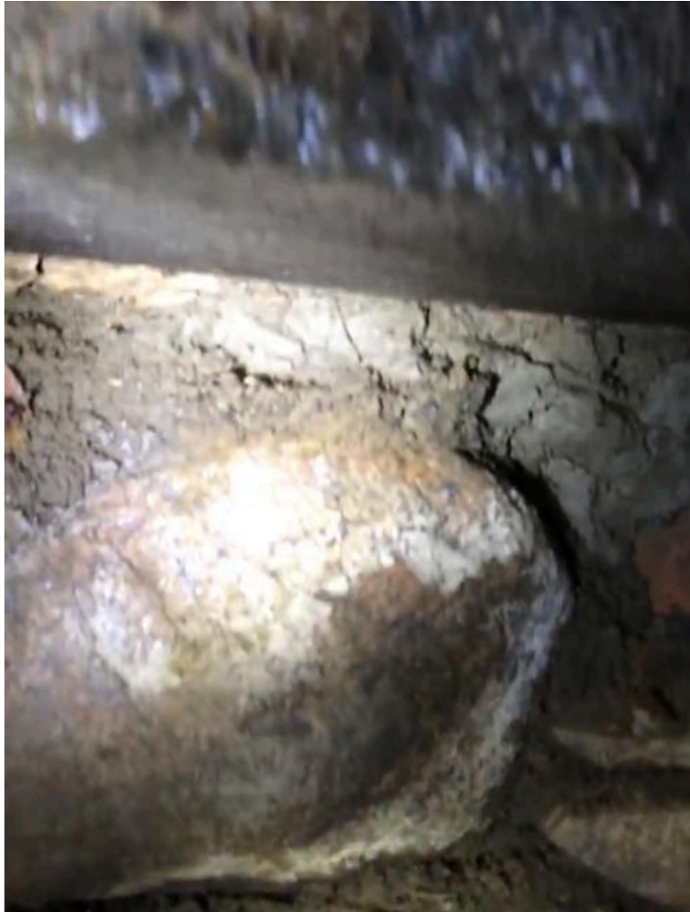
Figure 27- Well cap (top) and stones of well showing only areas where mortar is used near the surface of the well. Width of view is approximately 1 foot.
