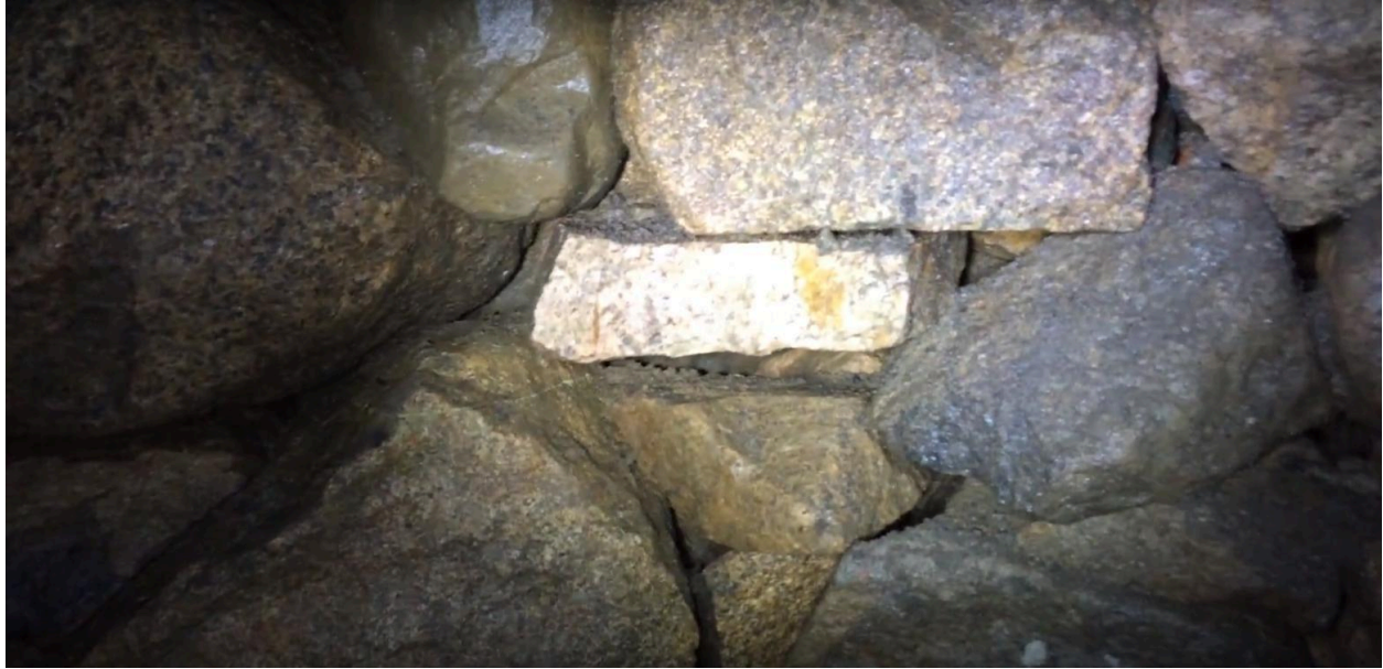
Figure 29- Video still showing stones in well structure. Note lack of mortar. View is approximately 2 feet wide.
