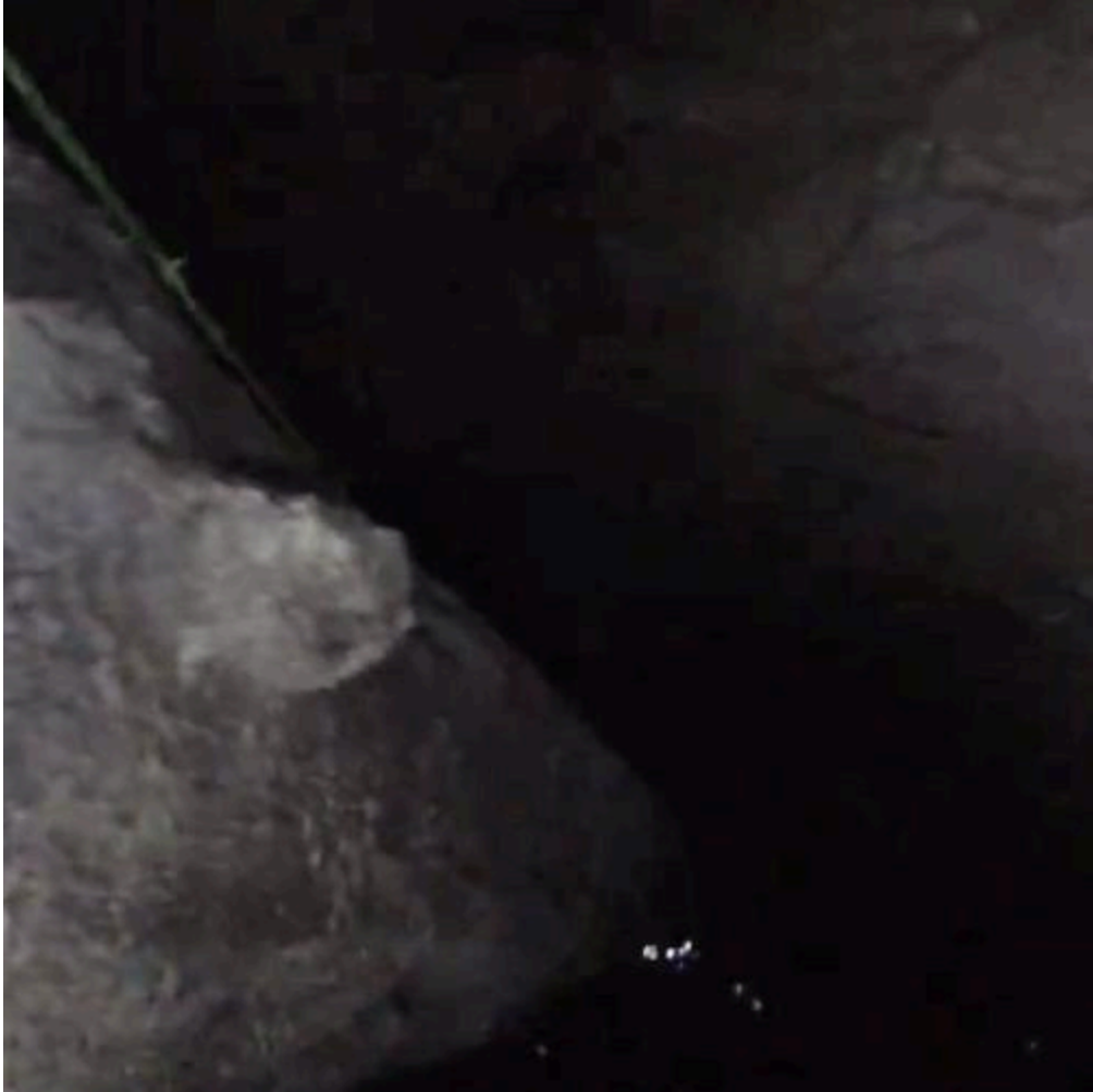
Figure 36- Possible remnant of a branch on exterior of pipe. Pipe is approximately 10 inches wide. View facing downward.
