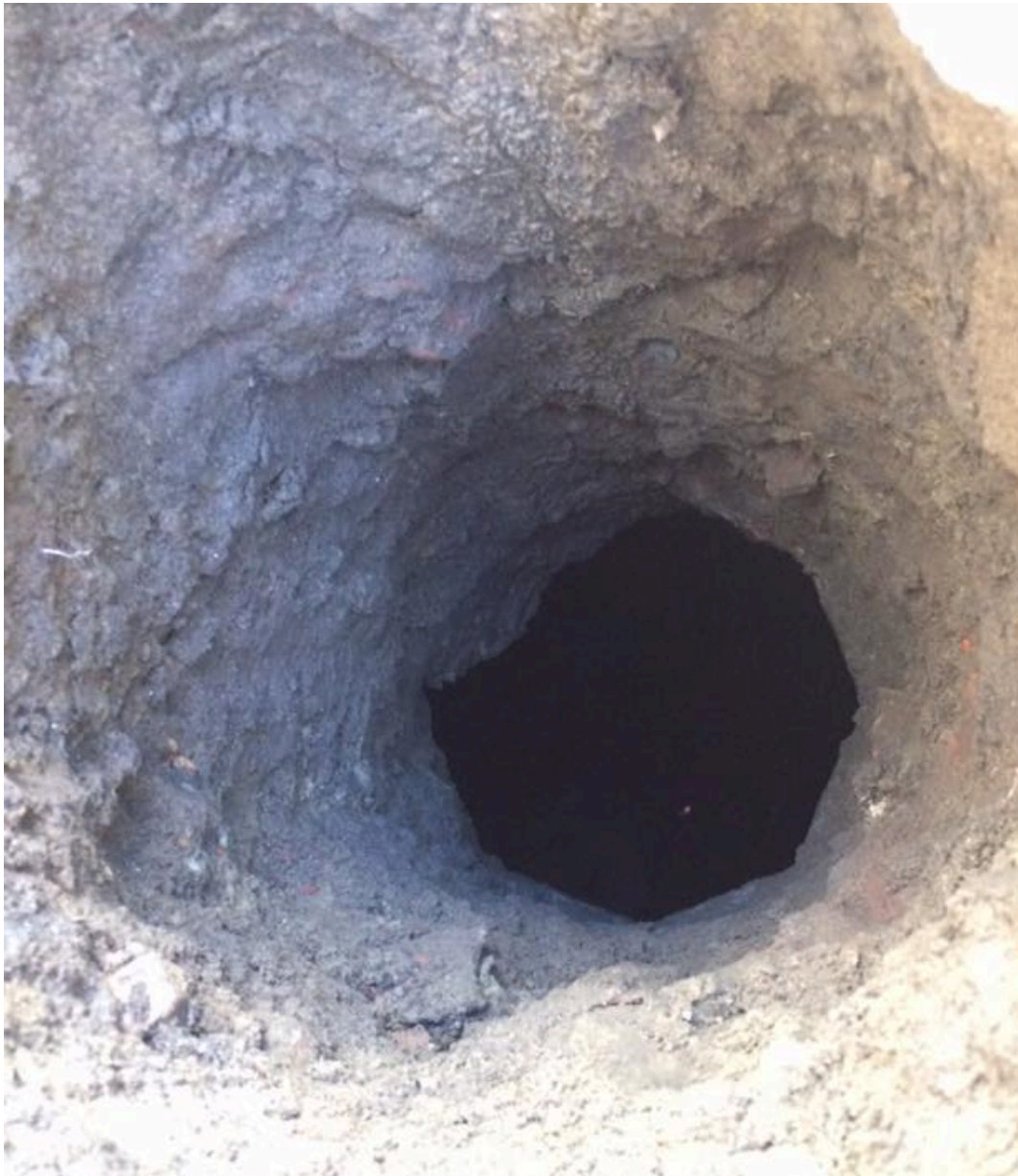
Figure 20- View pointing straight down from the surface of the opening of well. Octagonal opening is 12" wide (30 cm). Note consistent sandy fill above the opening. White dot in black void is the sun-lit octagonal opening reflected in water at the bottom of the well.
