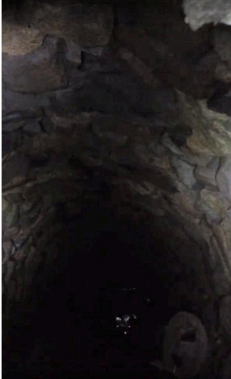
Figure 28- Video still of the well shaft just below the well cap. View shows pump pipe in the lower right. Width of view is approximately 4 feet.
