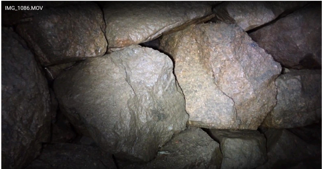
Figure 30- Video still of interior wall of well showing materials used in its construction. View is approximately 2 feet wide.
