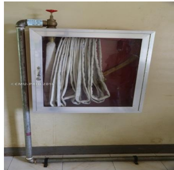
Fire box with dry stand pipe
