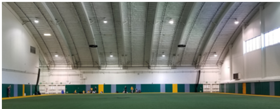
Figure 3: Field House area looking west with existing lighting fixtures (Pham 2019).
