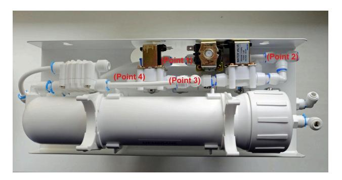
Will put the pressure sensor at the point 4 and replace the water supply pipe to the membrane. Connect a control loop.
