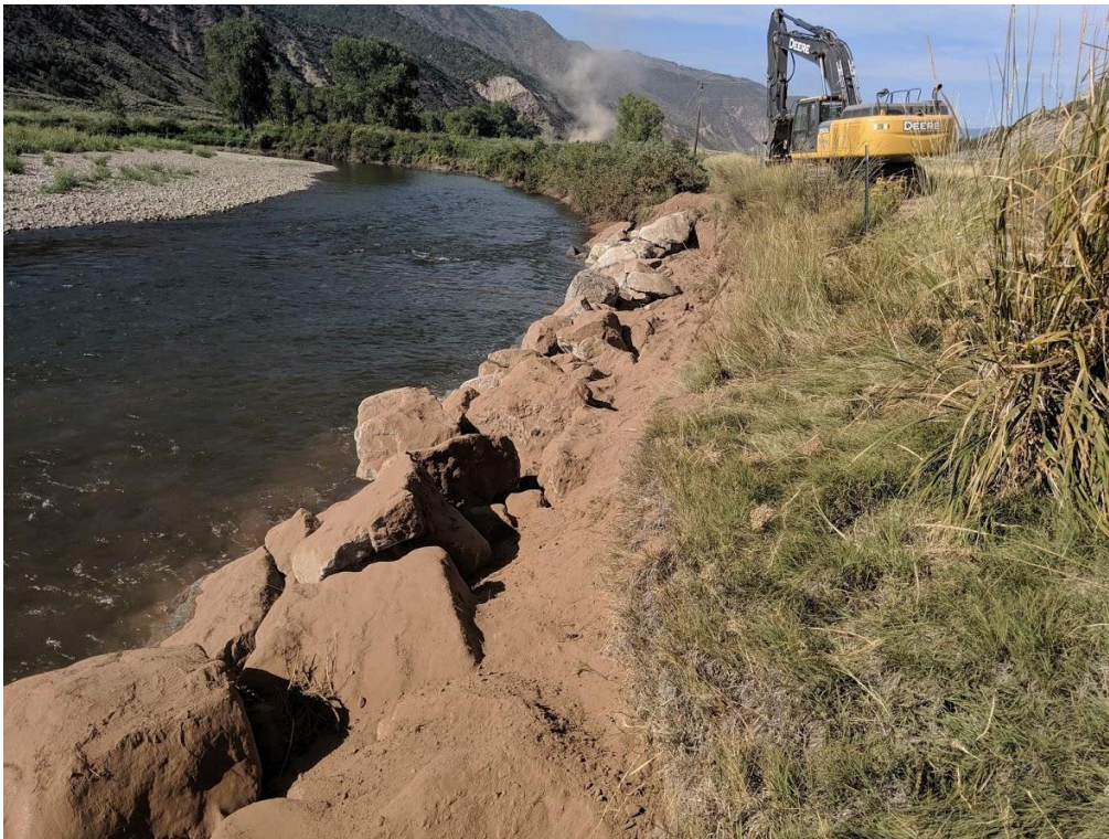
Figure 1: Riverbank Armor Installed in 2019.
