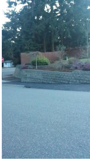
Image Showing: a retaining wall in my neighborhood
