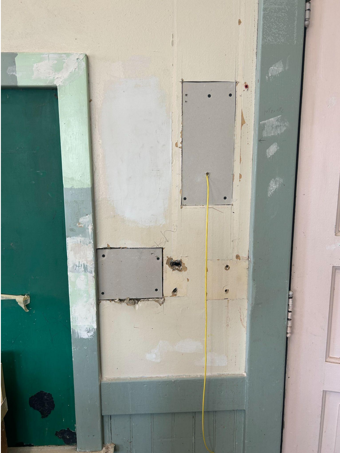
The framing contractor is going around and sealing up holes that were made in the existing walls or where electrical devices were removed.
