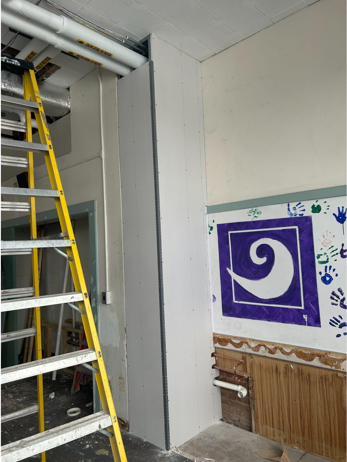
The piping and electrical conduits are being covered up by new chases being installed by the framing contractor.
