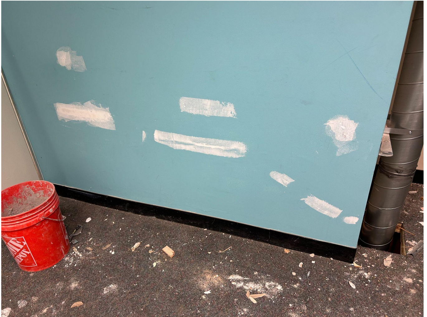
Sheetrock mud is being placed on the walls to cover up holes that were made during construction.
