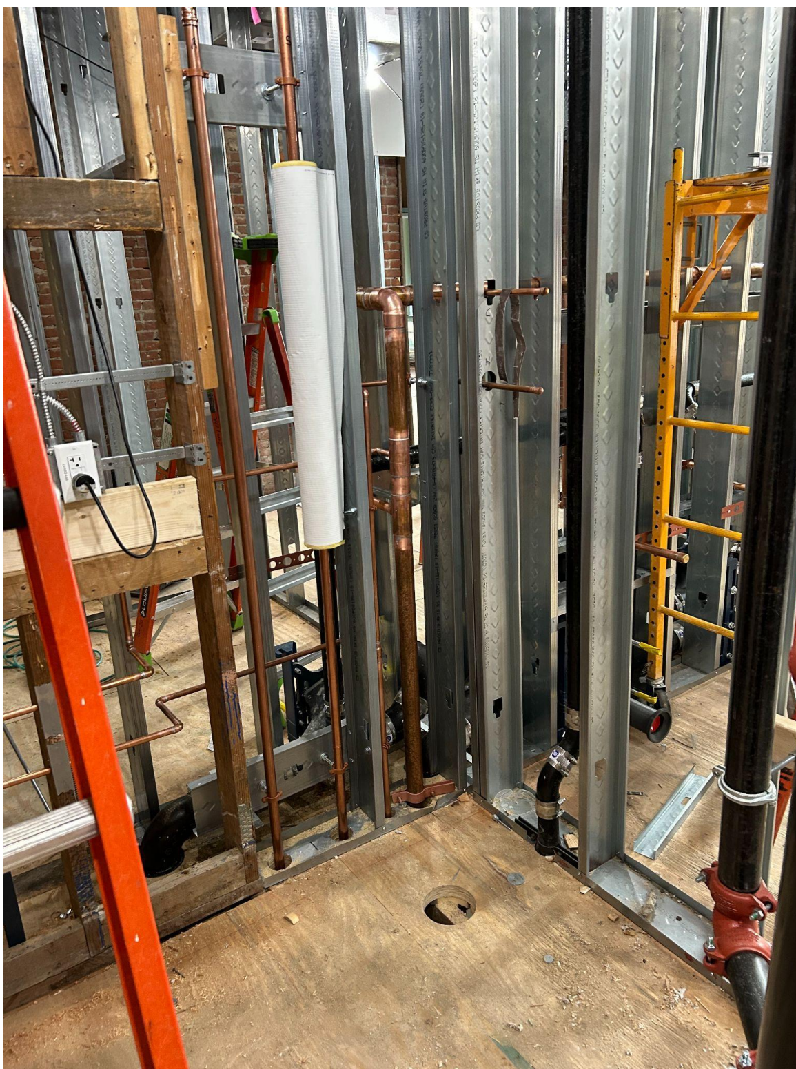
The installation of the copper piping for the gang bathrooms on the second floor in the 1904 wing of the building. The copper piping is for the domestic cold and hot water piping to the fixtures.
