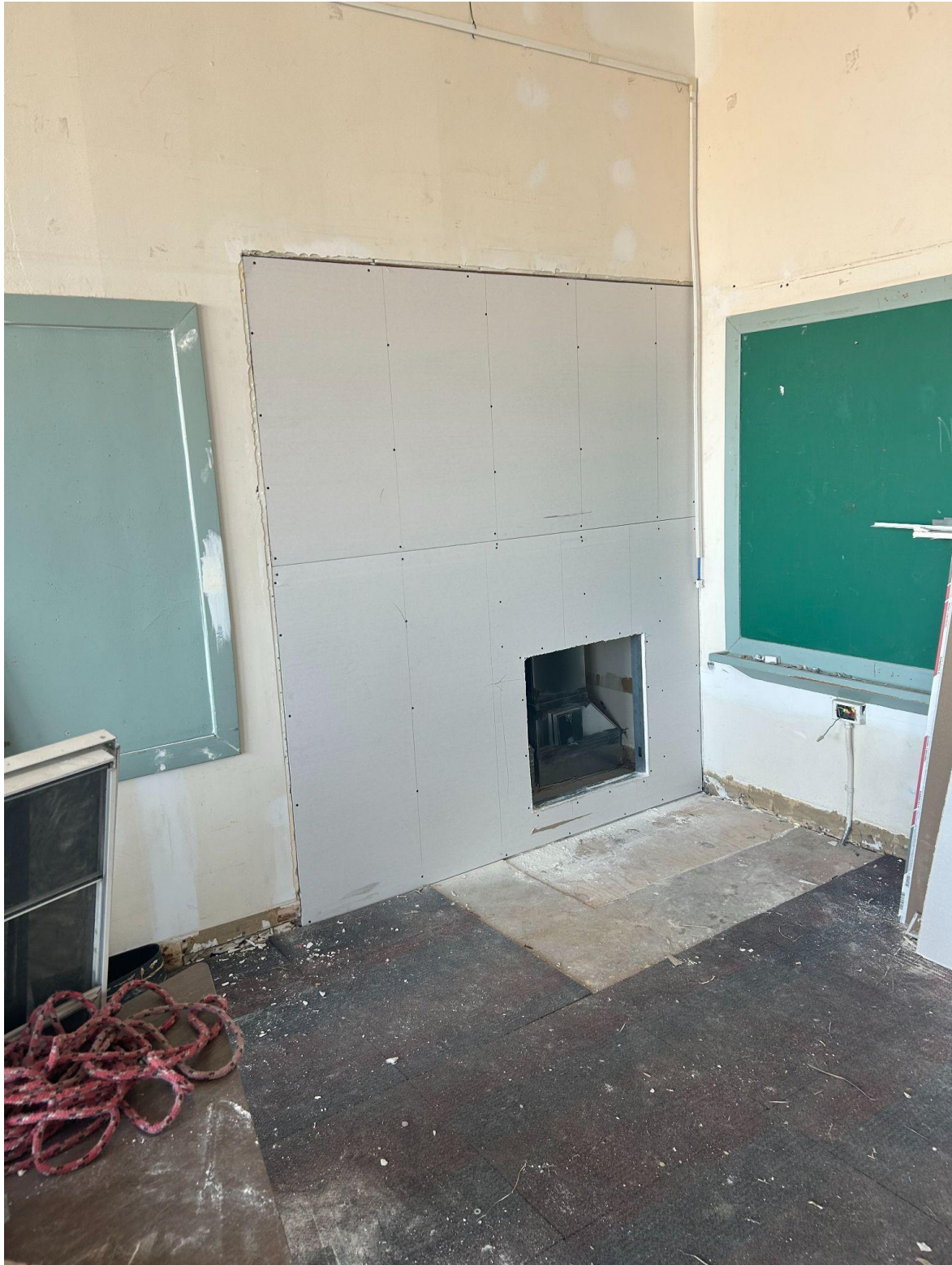
Another area where the framing contractor is covering up where ductwork, sprinkler piping, electrical conduits from one floor to another are getting covered up.
