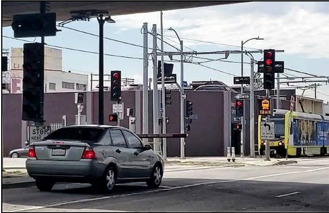
Figure 6: LA Metro left turn gate
