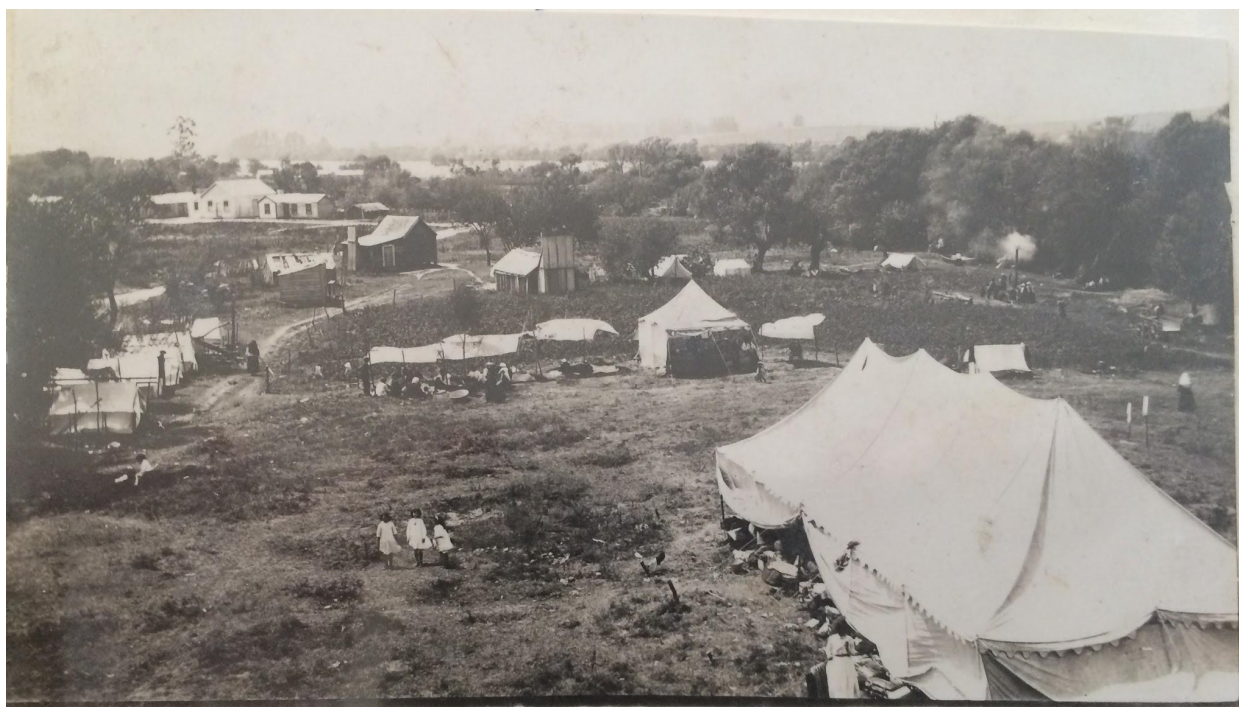
Another view of Thitar grounds at Korongata N.Z.
