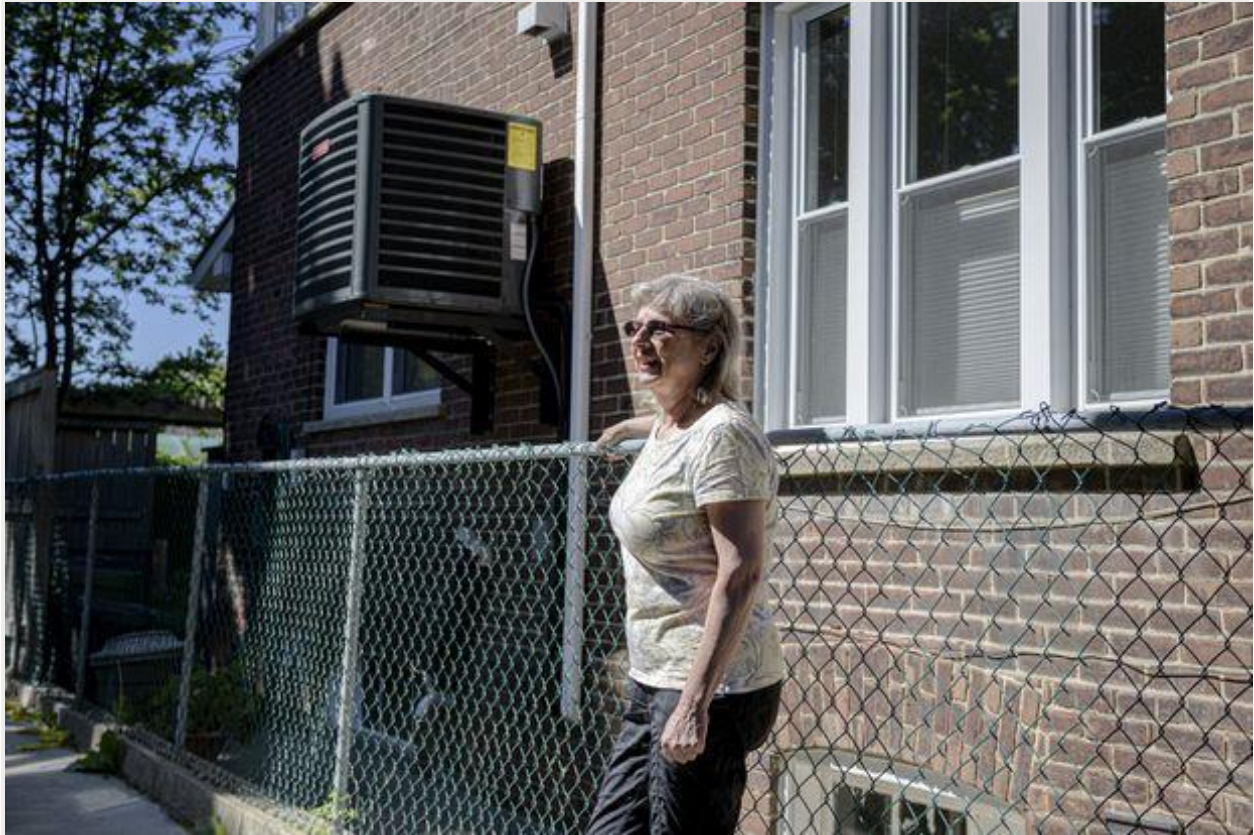
Ms. Wyatt next to the heat pump unit installed outside her home.
