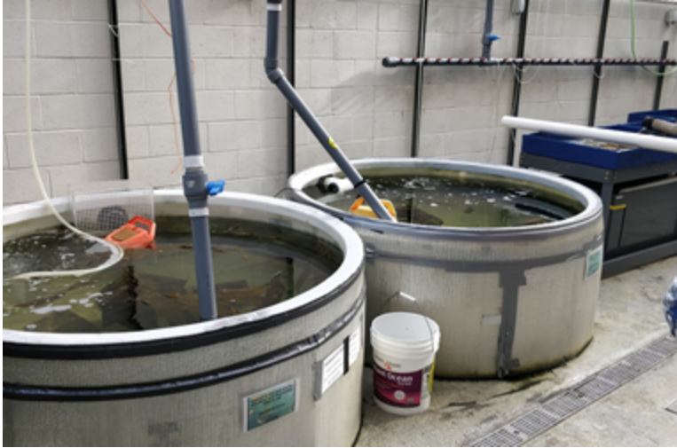
Figure 1: Outside tanks w/air rail
