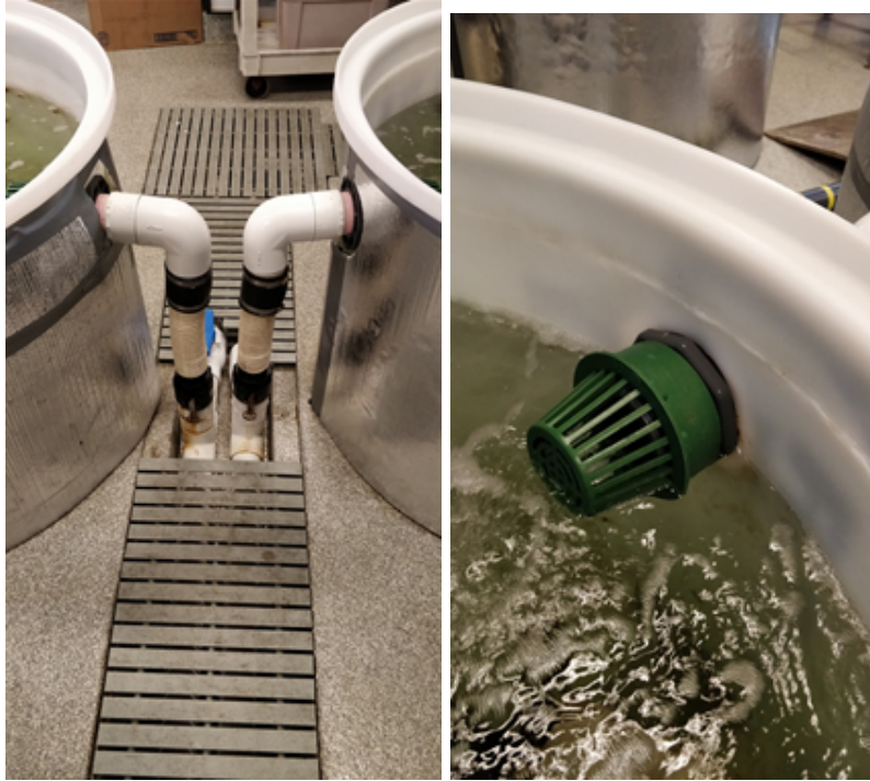
Figure 4: Tank Drainage pipes Figure 5: Drain inlet from tank
