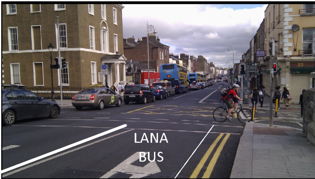
Fig 18 Single lane entry and exit outbound with two lanes on Ranleigh Bridge - convert to Bus lane and Cycle lane
