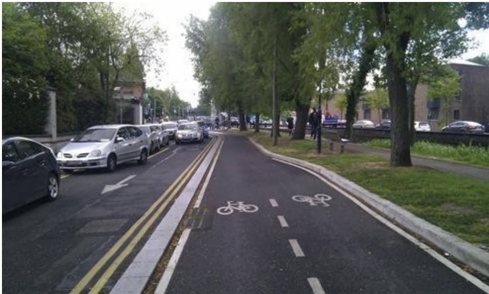
Fig 3 - quiet section of Canal Cycle Track mid morning...also notice track narrowing due to trees and preservation of parking on adjoining service road.
