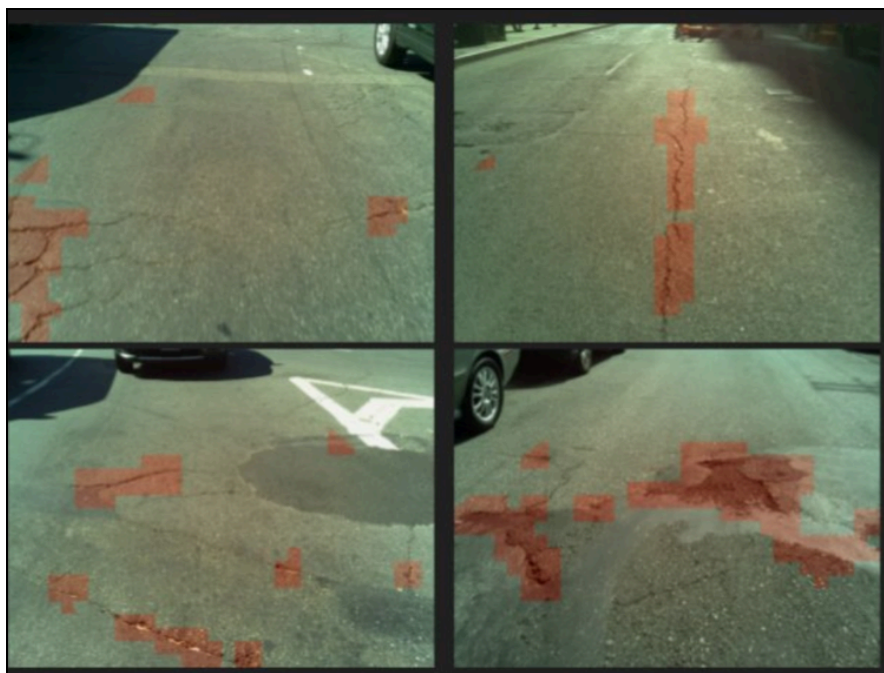
Figure 6: ARGO's computer vision model built on a training set of 100,000+ images of street quality. This model automatically detects large street defects using high-quality street imagery.
