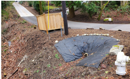
Photo 3: Black tarp around a pipe
