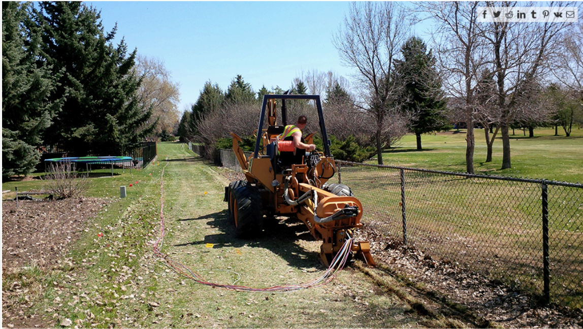
Connaught Subdivision: Irrigation Installation
