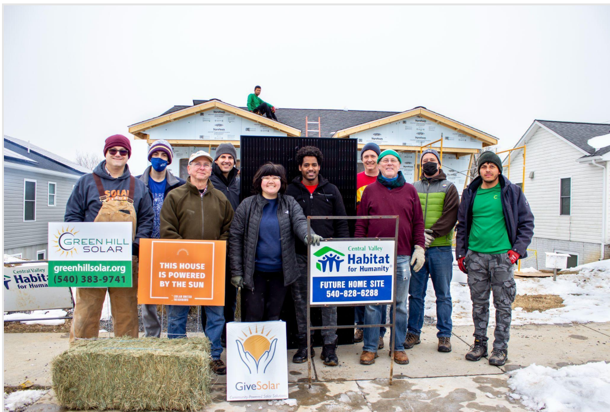
Solar barn-raising volunteers in Harrisonburg, Virginia, on January 28, 2022.
